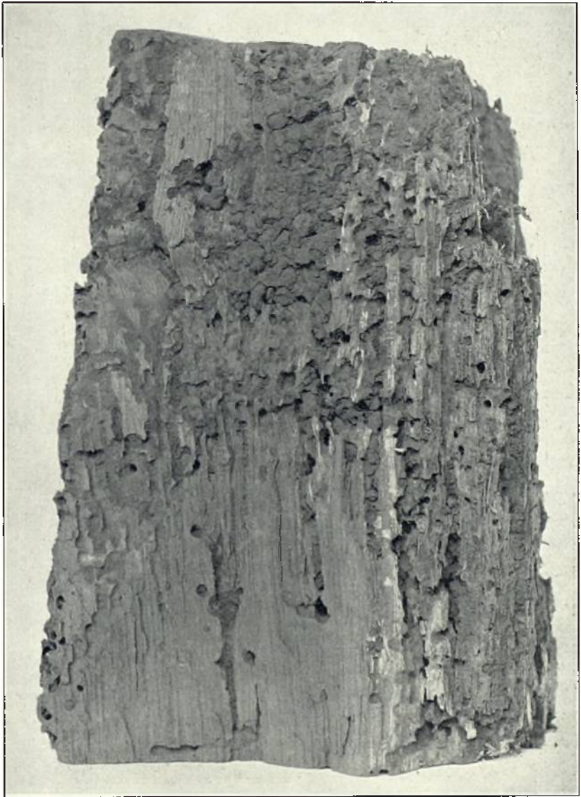
Portion of oak beam showing damage by Xestobium rufo-villosum .
