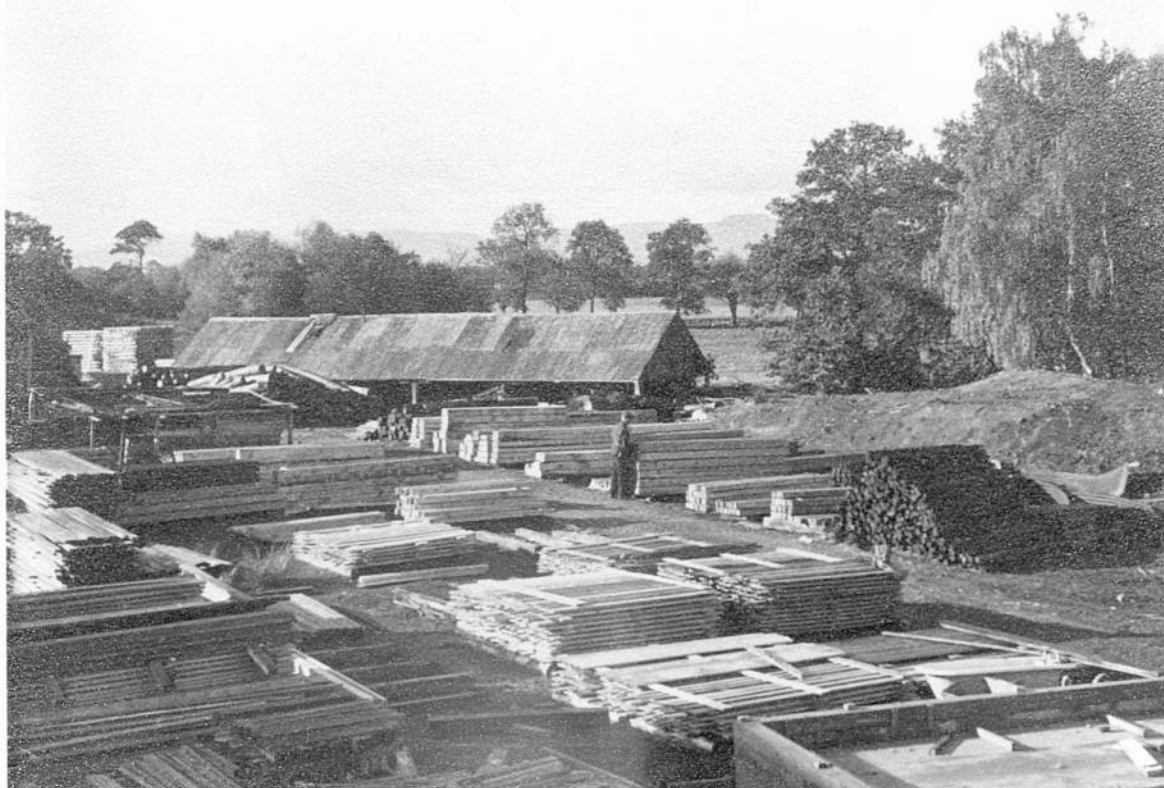
Culloden Sawmill provides Fencing material, Huts, Offices, Stables etc. for most of the needs of the Conservancy.
