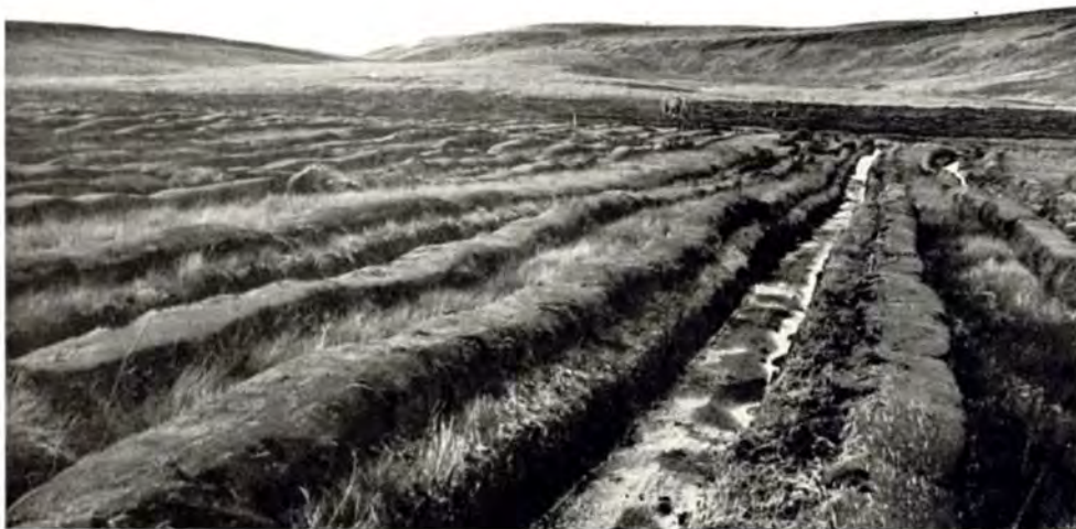
PHOTO 7. Strathy Forest, Sutherland, 1950. Deep Scirpus peat ploughed with the double mouldboard Cuthbertson plough, cutting furrows at 10 feet apart and spacing ridges at 5 feet.
