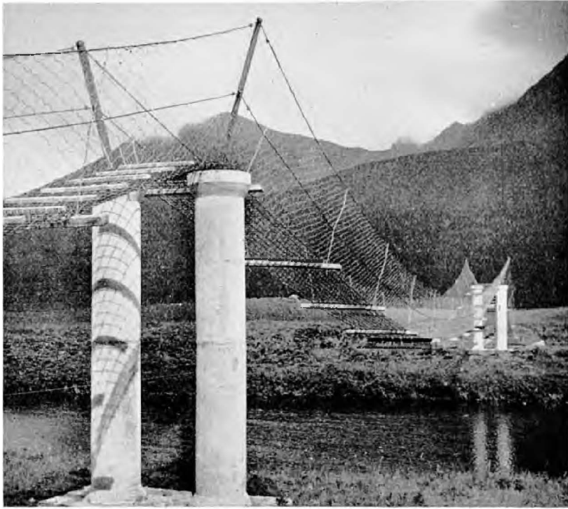
Photo 6. Wire-mesh suspension footbridge at Glen Brittle Forest, Isle of Skye.
