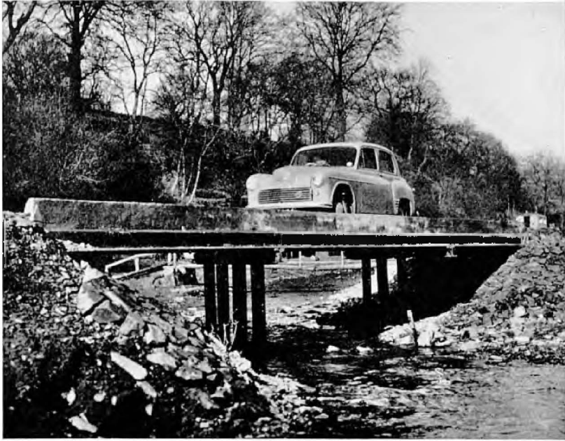
Photo 8. Forest road bridge constructed with tramrails.
