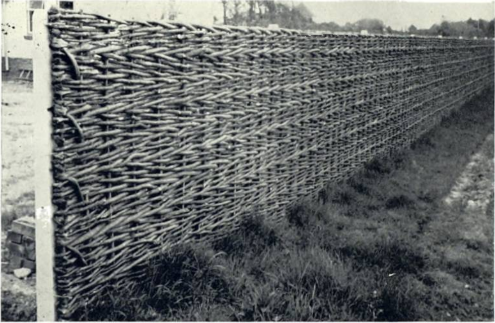
Plate 26. Detail of continuous round-rod wattle
