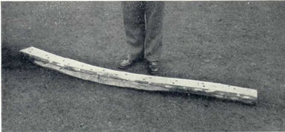
Plate 16. Typical "break" for hurdle making. Note curved outline, and double series of holes for uprights to allow variation in spacing
