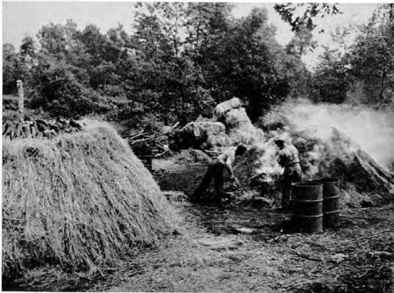
Photo 24. Charcoal burning. Left: A completed stack protected with straw prior to covering with earth. Right: A stack has been reduced to charcoal, about to be uncovered.
