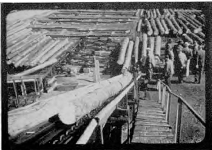
Plate 3. Begley: Mechanical sorting and handling of saw logs at Nangwarry.
