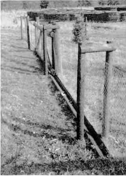
Plate 17. Small, Creosoted Sliding Gate: Arrangement of split rail runners at ground level, forming a groove for easy sliding.
