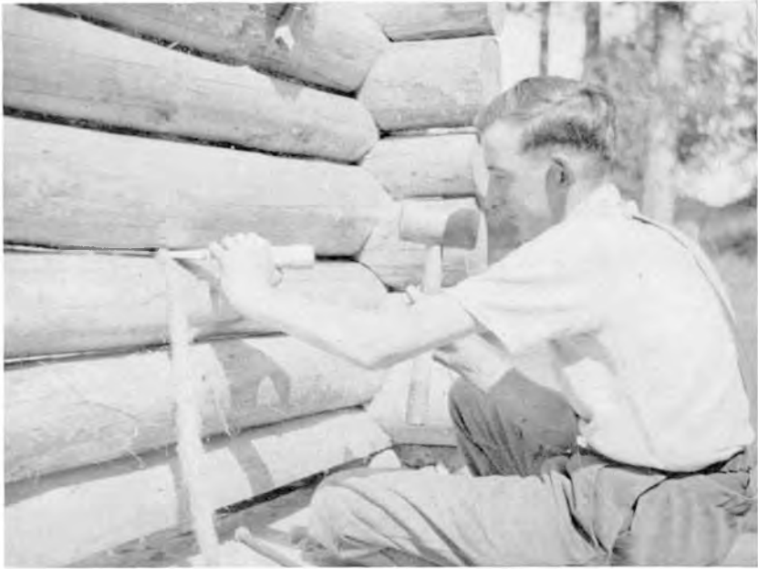
Plate 15. Watson, Log Chalet: Caulking with rope.
