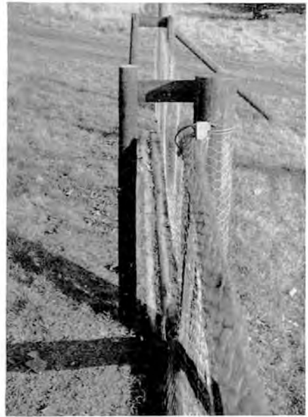
Plate 20. Small, Creosoted Sliding Gate: Close-up showing close fit of gate to posts, essential to make it rabbit-proof; also iron hook used to keep it closed.
