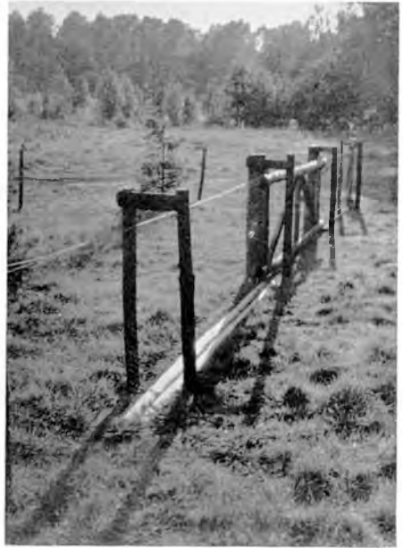
Plate 18. Small, Creosoted Sliding Gate: Alternative use of peeled poles as slides.
