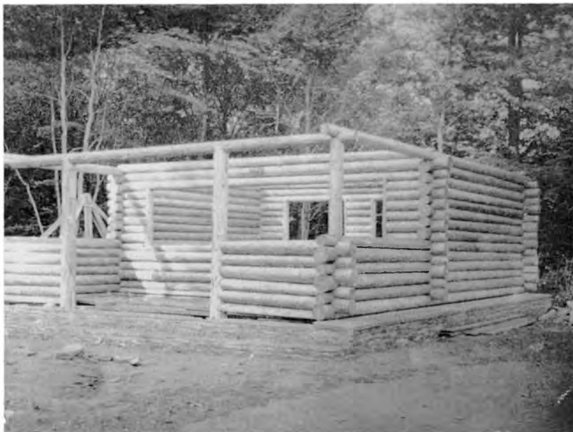
Plate 13. Watson, Log Chalet: The building finished to wall height.
