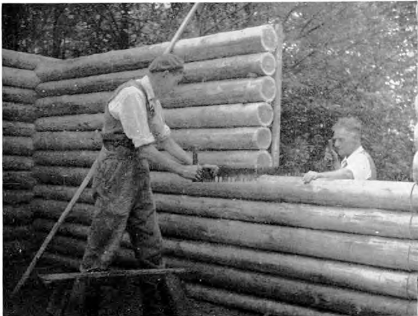
Plate 12. Watson, Log Chalet: Cutting a door opening.
