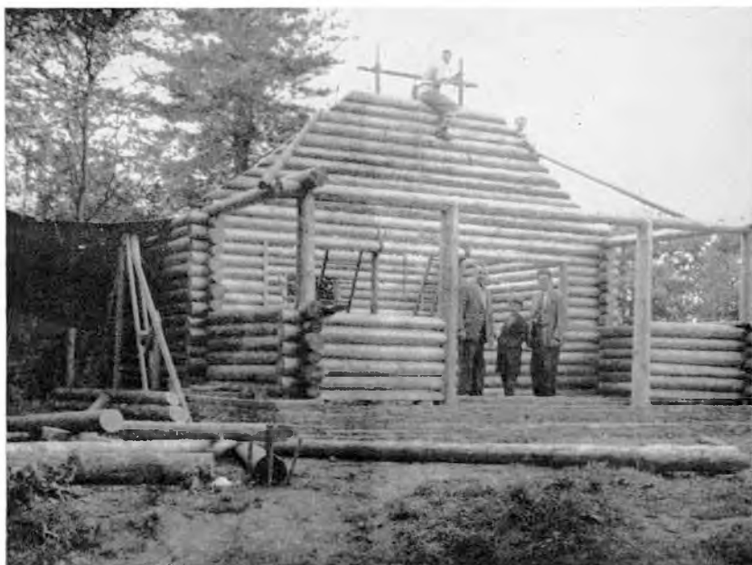
Plate 14. Watson, Log Chalet: Building the rear gable.
