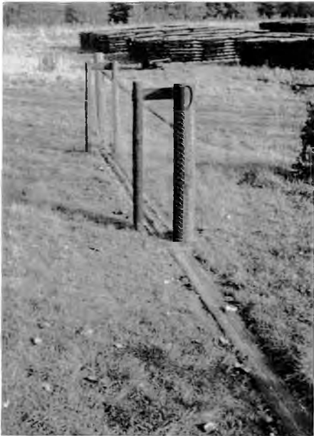
Plate 19. Small, Creosoted Sliding Gate: Flat sill at ground level.
