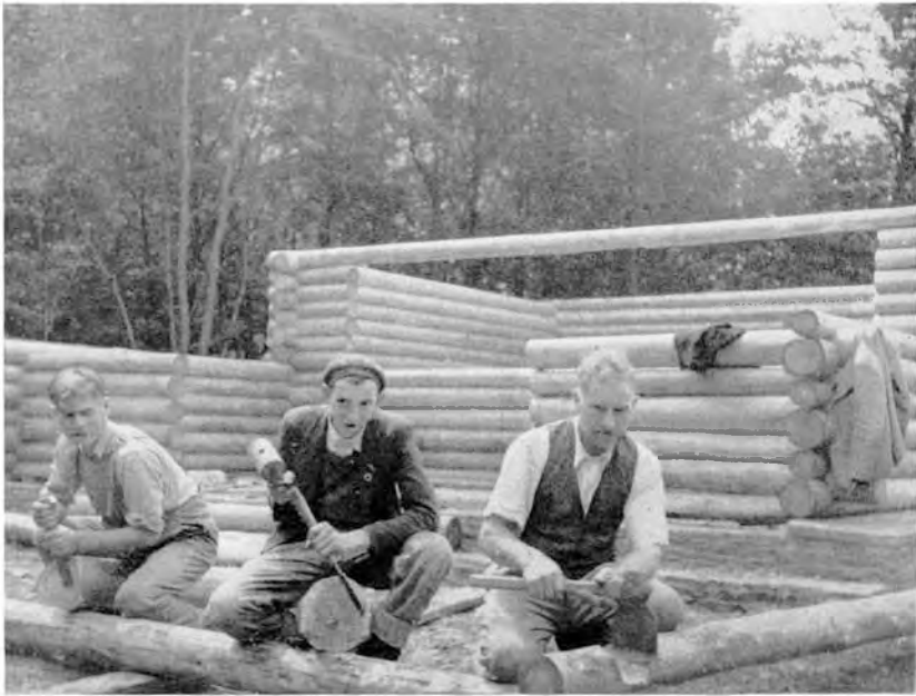
Plate 11. Watson, Log Chalet: Notching the Logs.
