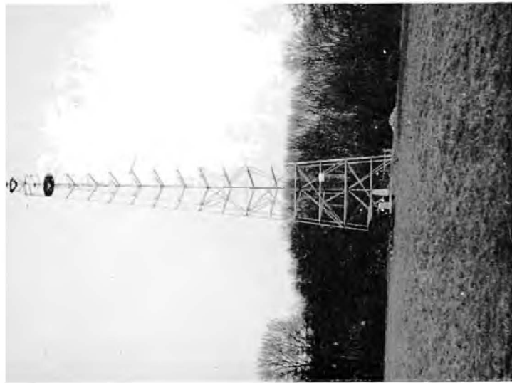
Plate 8. Bilby Steel Tower, used by the Ordnance Survey to take bearings over flat country; theodolite isolated in centre, to avoid sway.
