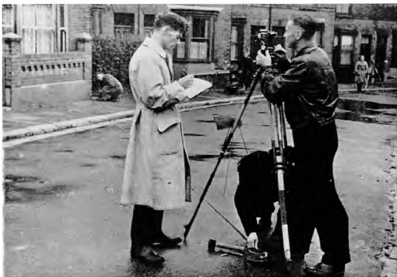
Plate 11. Survey party fixing Revision Points, as a basis for final stages of chain surveying.
