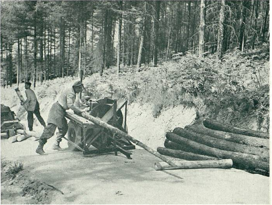
PLATE 4. Peeling and cross-cutting pitprops at Dalby, Allerston Forest, Yorkshire.
