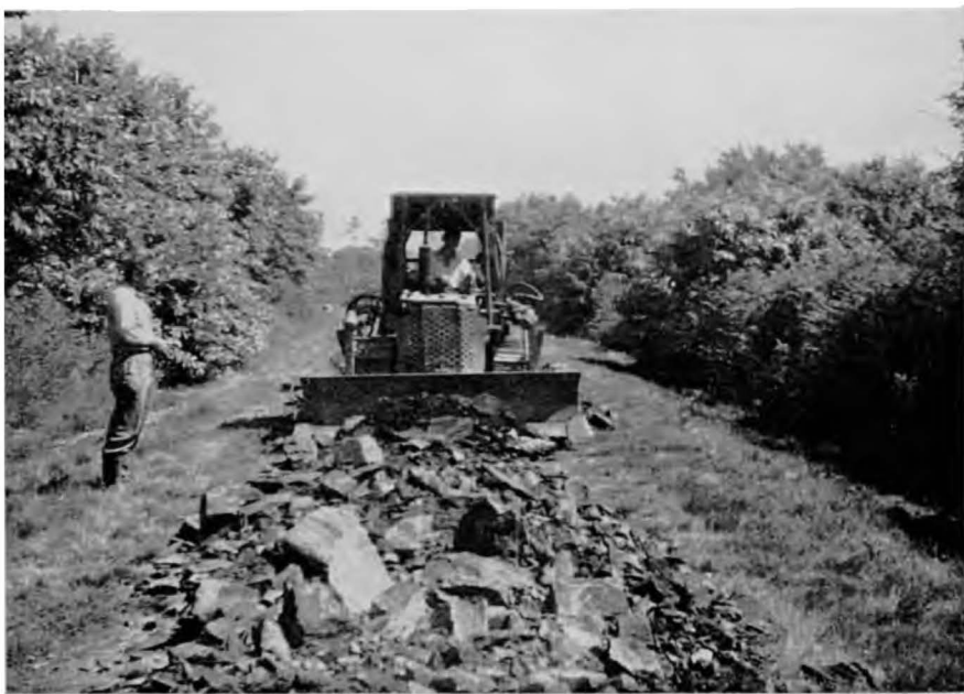
Plate 11. Road-making, Lyminge: The bulldozer spreads the shale.
