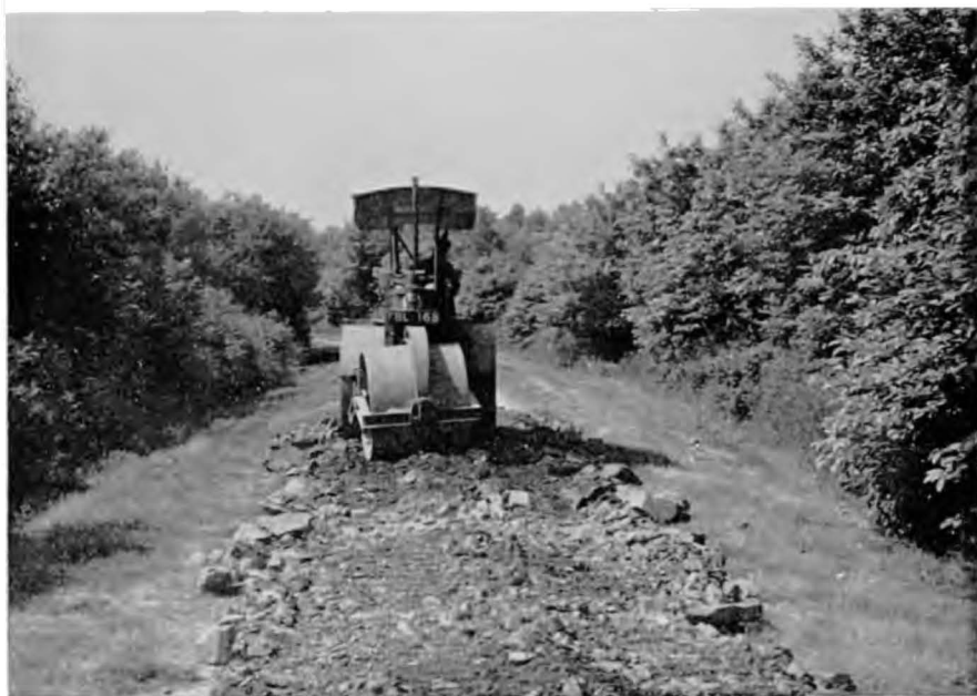
Plate 12. Road-making, Lyminge: Diesel roller compacting spread shale.
