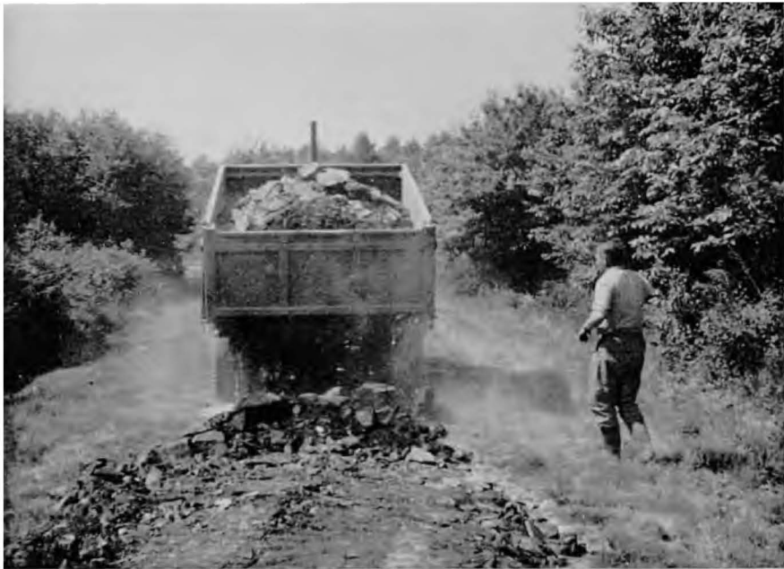
Plate 10. Road-making at Lyminge Forest, Kent: Tipping the shale.
