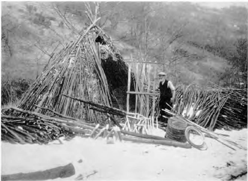
Plate 5. A Dean Craftsman, about 1925. He made hurdles, chair legs, and barrel hoops. His round hut, built of poles and thatched with wood shavings, is built on a plan unchanged since Neolithic times.
