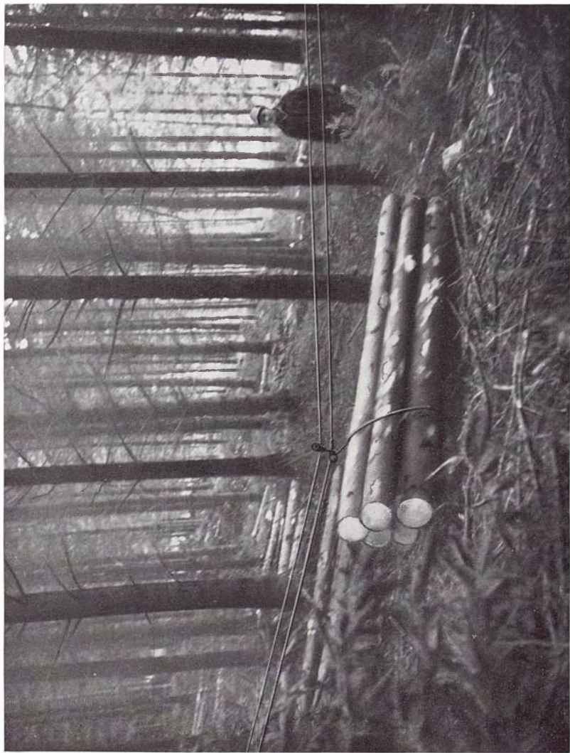
PLATE VIII The choker man stands clear as a load starts. Note his hard hat.
