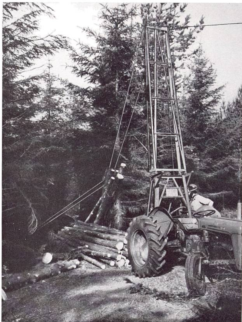
PLATE II General view as a load reaches the stack.
