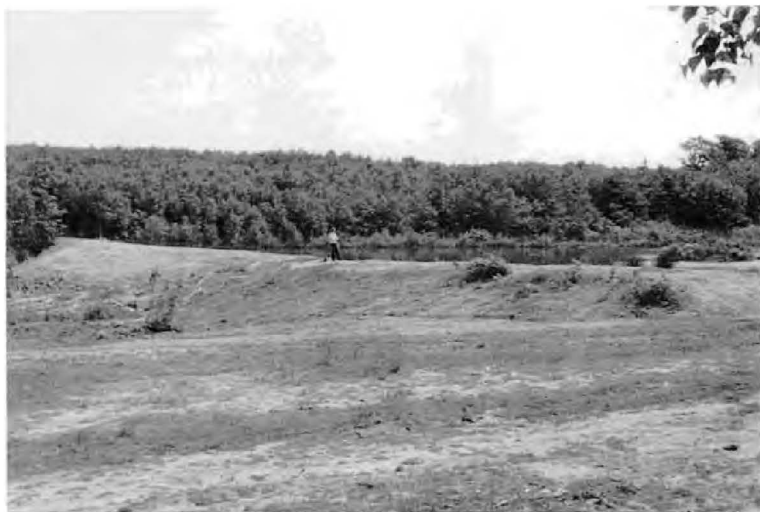
PLATE 20: Abbot's Wood Pond at Friston Forest, Sussex. After recent improvements the pond is now used as a source of water for fire-fighting and as a wild life sanctuary.
