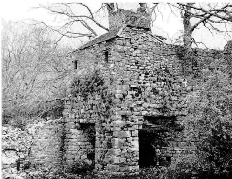
PLATE 7: A remarkable relic of a forgotten forest industry. This furnace on Loch Awe-side, near Taynuilt, used charcoal from the Argyllshire oakwoods to smelt iron ore in the early nineteenth century. Contributed by Tom Weir, well-known climber and photographer.
