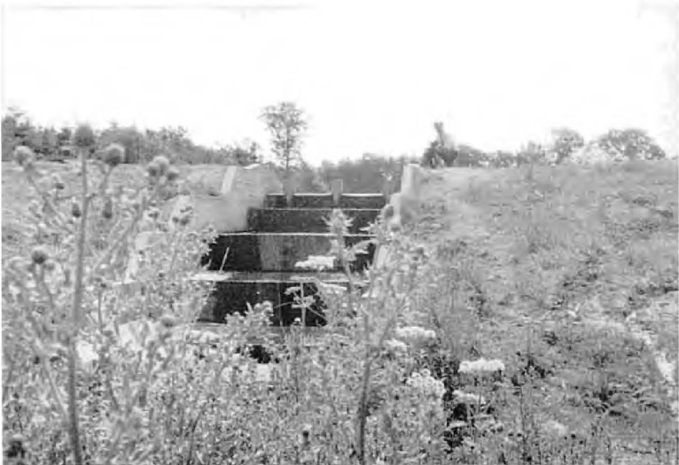
PLATE 23: The spillway at Abbot's Wood Pond.
