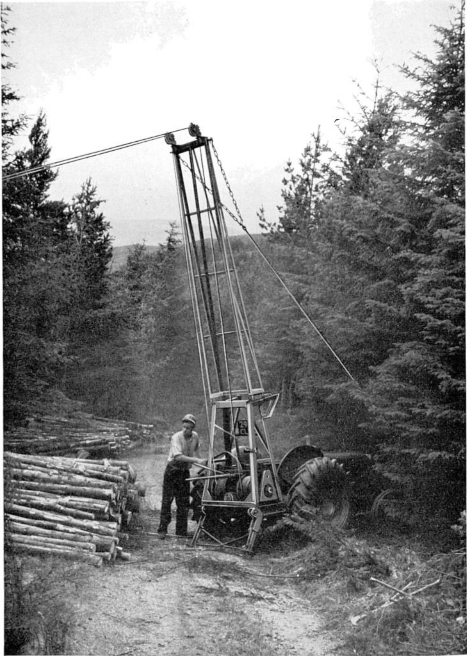
PLATE 10. Zehetmayr, Work Study, and Shaw, Machinery Research: General view of Norwegian Isachsen Double Drum winch. Note drums at rear of tractor, and two hauling lines at head of tower.
