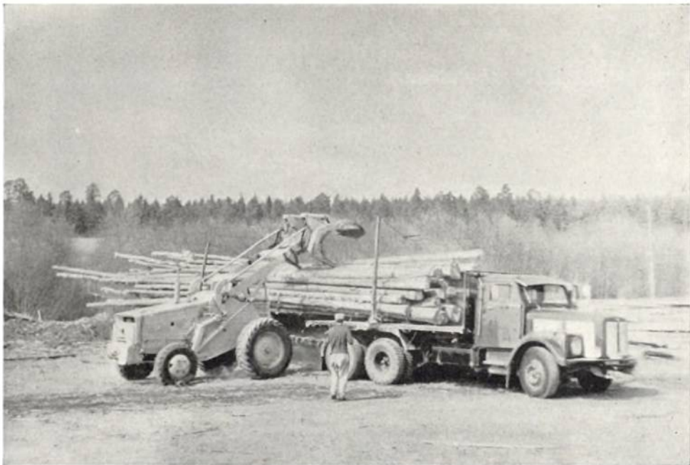
Plate 35. A Bolinder Munktell (B.M.)-Volvo 225 tractor equipped with hydraulic grab unloading 40 feet to 50 feet poles from a pole wagon at the log handling depot of Wistavarfs A.B. near Sundsvall. The weight is transferred to the large driving wheels—which are the front wheels of the tractor when used for this purpose. (The driver faces backwards and it is driven backwards. It is equipped with an excellent safety cab.) A similar tractor was used by the Swedish Cellulose company to feed trees to the Sund barker.
