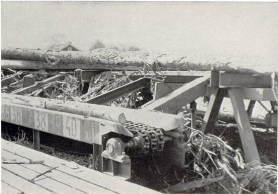
Plate 37. The beginning of the single line conveyor belt. One tree length at a time is moved forward mechanically—by push-button control—to the conveyor belt.
