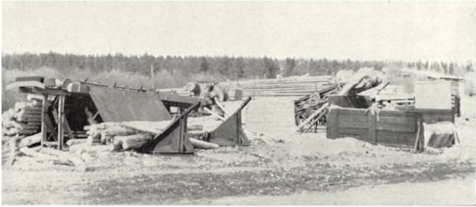
Plate 42. The end of the production line at the log handling depot of Wistavarfs A.B. near Sundsvall. Cambio barker in centre of picture—with conveyor belt removing bark to a clearance bay on right. Note that each side of the end of the single line conveyor belt is a steel cradle—one on each side. The near cradle collected pine pulpwood; the remote cradle collected spruce pulpwood. Pine and spruce sawlogs had been kicked off to either side in similar fashion before reaching the Cambio.
