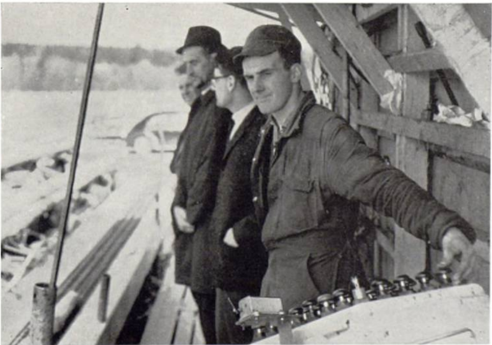
Plate 38. The push-button control box. The two engineers who designed this equipment are standing behind the controller. The single-line conveyor belt is on the left.
