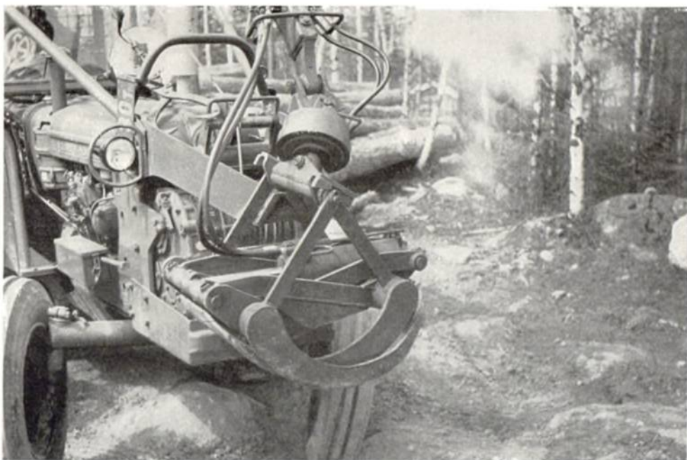
Plate 8. The Osa hydraulic grab with horizontal piston, which saves about 18 inches in height.
