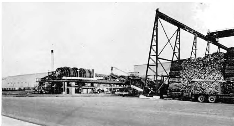
PLATE 21. A general view of the new Thames Board Mill at Workington, Cumberland, opened by Mr. Harold Wilson, the Prime Minister, on 9th June 1967. Stacks of un-barked poles are seen on the right, with the de-barking drums on the left; a conveyor system links the two.
