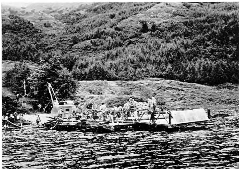
PLATE 20. Landing the excavator, from the specially built pontoons, at Glen Hurich. Photos contributed by Mr. J. V. Dishington of the Engineering staff.
