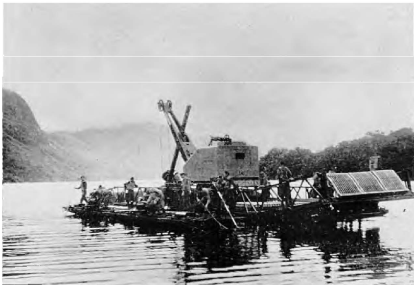
PLATE 19. Royal Engineers rafting a Priestman Cub excavator down Loch Shiel for the construction of the new Commission road from Glenfinnan to Glen Hurich Forest in Argyll. The excavator, weighing twenty-four tons, was floated for six miles down the loch, during the summer of 1962.
