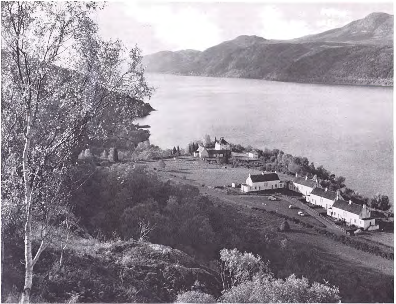
fig 33 Forest Workers' houses at Farigaig Forest above Loch Ness in the Great Glen of Inverness-shire.
