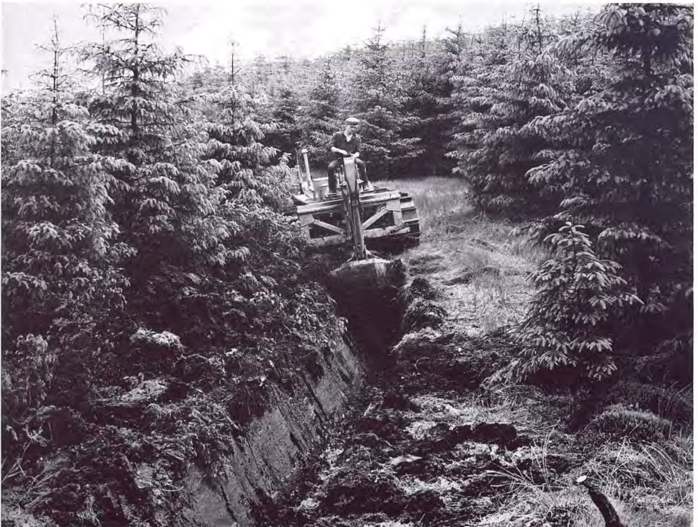
fig 37 A back-acting digger deepens drains to improve root growth and stability in a crop of Sitka spruce at Carron Valley Forest, Stirlingshire.
