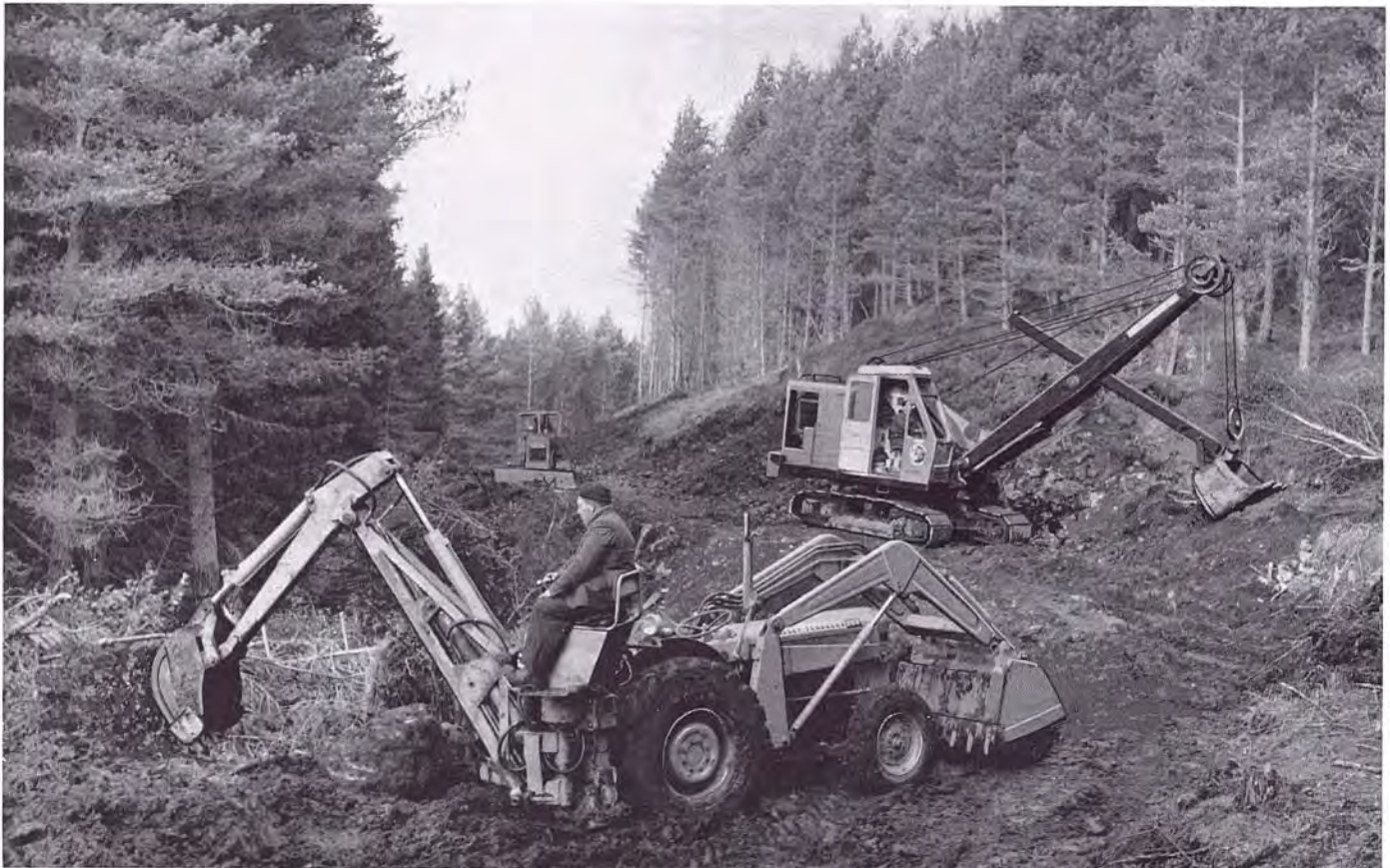
fig 28 Heavy construction machinery excavating a road formation in a Highland forest.
