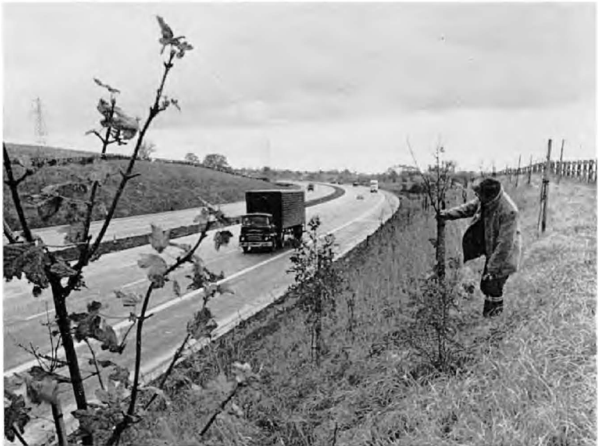
PLATE 9. Larger trees, requiring staking, are planted along a cutting. Besides improving scenery, both these measures will lessen wind pressure on cars and vans, leading to safer steering at motorway speeds.
