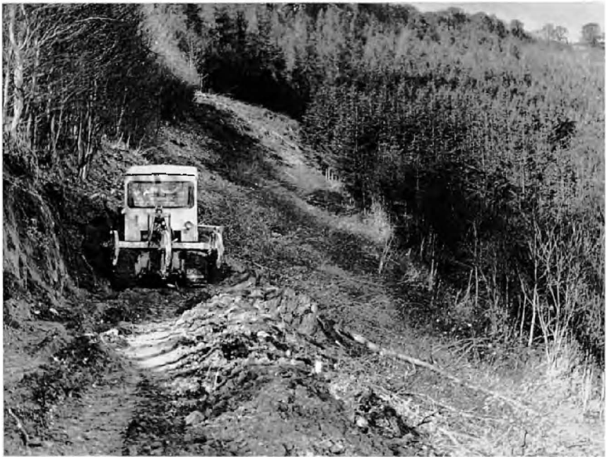
PLATE 15. A bulldozer excavating the road-bed for a new forest road along the steep Greensand slopes of Monkton Wyld Wood, in Charmouth Forest, Dorset.
