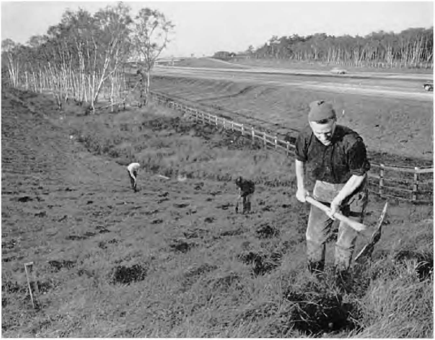
PLATE 8. Motorway planting beside the M1 in the English Midlands. Establishing a plantation, using small trees, to screen an embankment.
