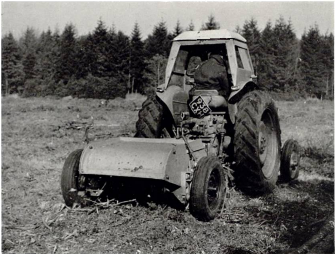
Plate 27. The Wilder Rainthorpe Scrub-Masta '40' flail-type weeding machine.
