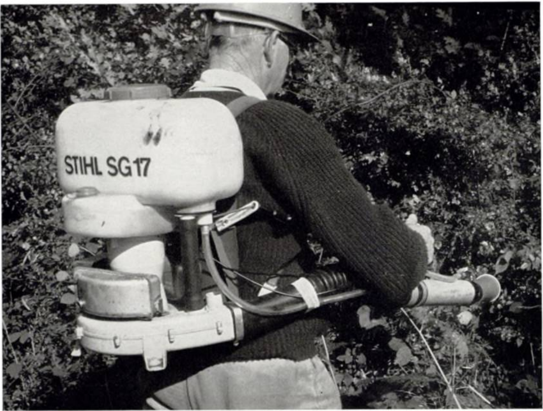
Plate 45. The Stihl SG 17 knapsack mistblower. WS 2/35/16
