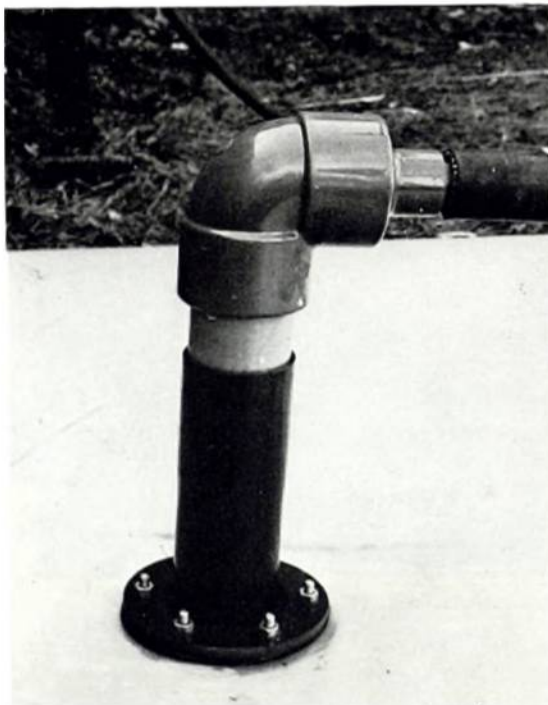
Plate 70. Detail of stack pipe and hose coupling. WS 2/6/14A
