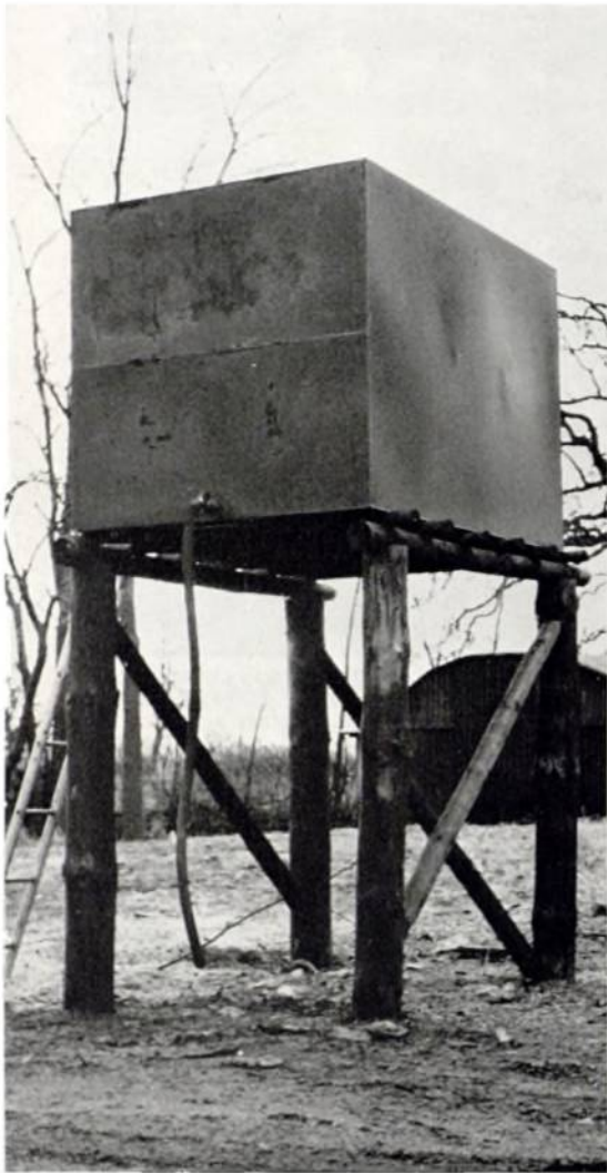
Plate 34. A 600-gallon (2728 litres) paraffin storage tank at Wymersley Forest (Northants). It is mounted sufficiently high to fill the transporting vehicle by gravity. WS 4/1/3
