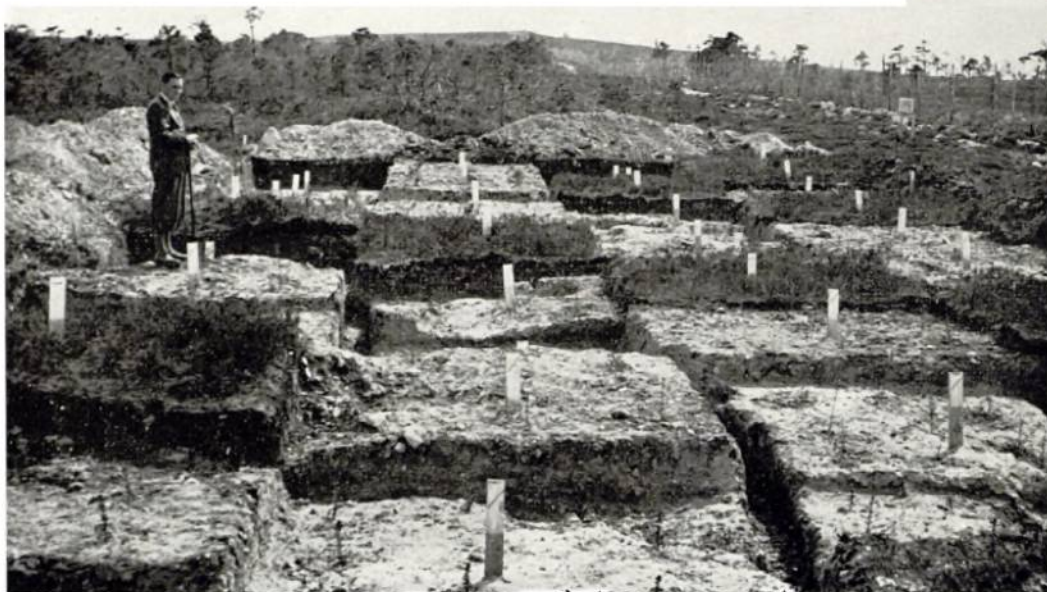
Plate 16. Method and position of planting experiment at Teindland, Laigh of Moray Forest, Morayshire, planted in 1934. Lodgepole pine, Scots pine, Japanese larch and Sitka spruce set into four different soil horizons: original surface, leached layer, pan, and subsoil. 1934. Ch. 5. C2160.
