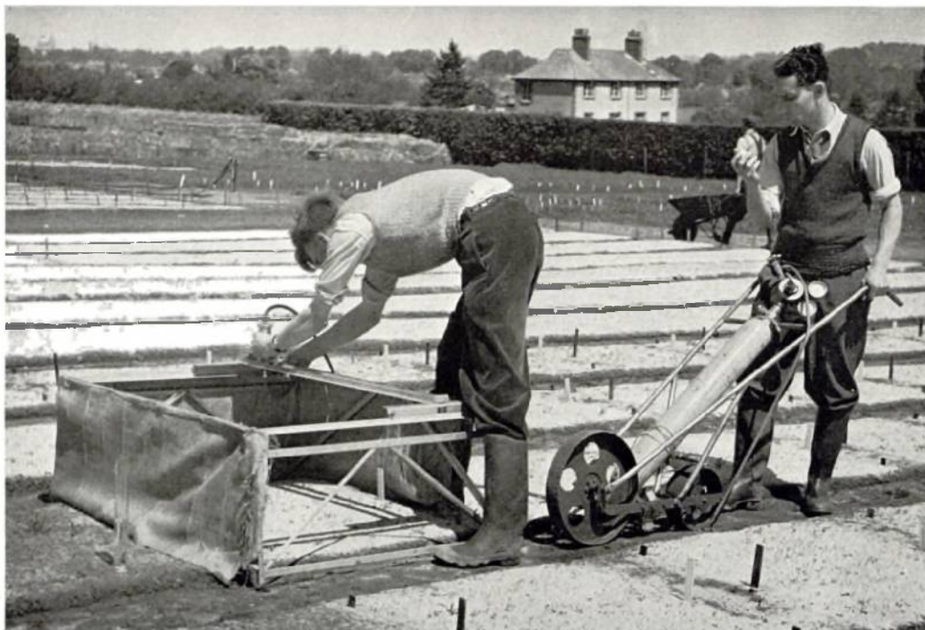
Plate 34. Nursery spraying of herbicidal oil at Kennington Nursery, Oxford, in 1950. The herbicide is put in the small glass container mounted on a traveller which traverses the plot in two directions at right angles. Air pressure is supplied from a fine pressure bottle and the herbicide emerges from a special jet on the traveller in a fine spray. Ch. 14. C76.
