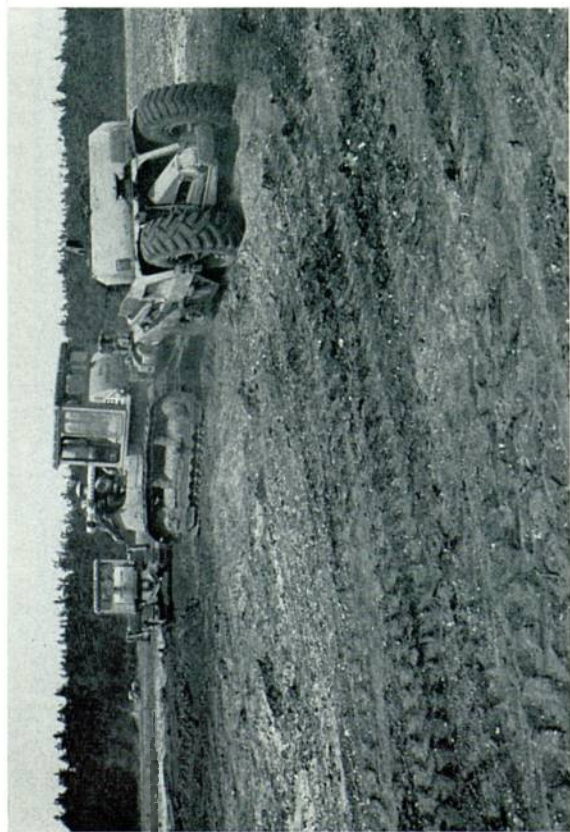
Plate 2—Site Studies South (p. 22). Gravel workings in Bramshill Forest, Hampshire. (above) Heavy machines used for grading restored land. B. 8776. (right) Multishank adjustable ripper used to relieve compaction by tining to 710 mm depth with a D8K tractor. B. 8777.
