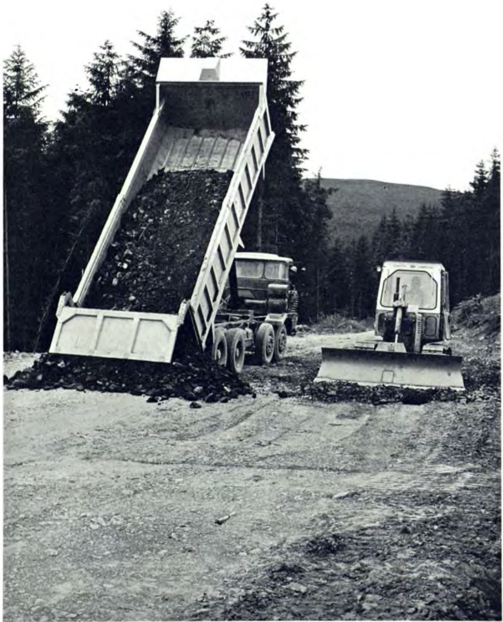
Plate 17 After widening the road formation to make a timber loading bay, the dozer spreads and consolidates the road metal delivered by tipping lorry. (p. 121).
