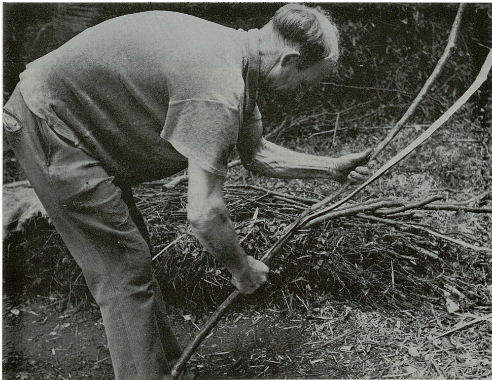
Figure 11. Hurdle making. Cleaving rods with the billhook.
