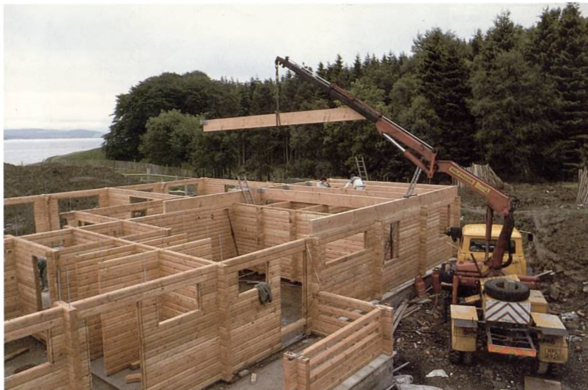
Plate 7. Construction – British Douglas fir used as beams in the construction of a visitor centre for the Northumbrian Water Authority by A.G. Stuart Ltd. (E8570)
