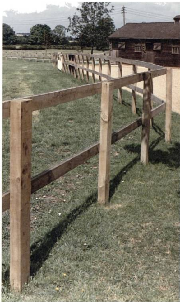
Plate 9. Fencing – Softwoods require treatment with preservatives to give a service life of 20 or 40 years. The post and rail fence round this paddock has been treated to the specification for 40 years. (Copyright: Building Research Establishment)
