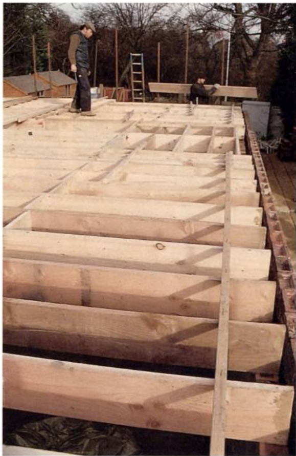
Plate 8. Construction – Machine graded Sitka spruce being used on a building site as joists in a suspended floor. (37933)
