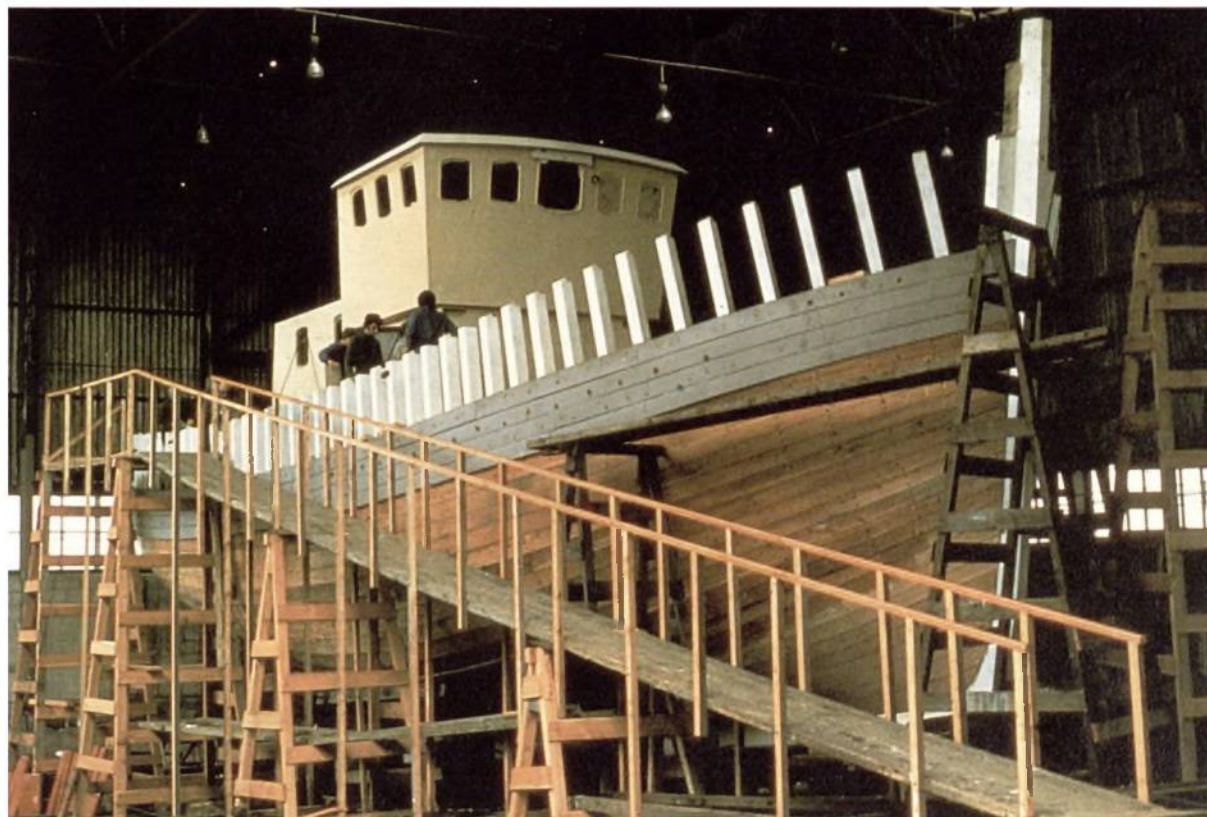
Plate 4. Boat building – Boatskin larch is required by this industry where skippers still specify wooden hulls for their fishing boats such as this one at Jones Buckie Shipyard Ltd. (E5919)
