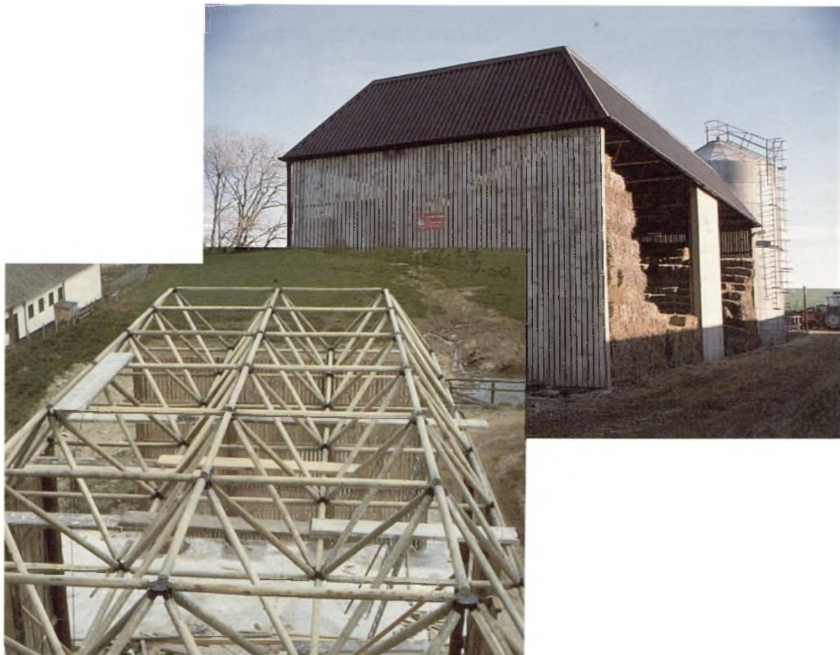
Plate 11. Farm buildings – A pole barn at Bridgit's Experimental Husbandry Farm near Winchester, designed by ADAS. (37729). The building was constructed using large treated round timber uprights and a novel system with short small diameter roundwood struts in the roof (Inset)
