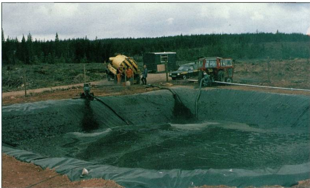
Plate 3 Storage lagoon constructed to hold sewage sludge before application to a restocking experiment on heathland at Teindland (Grampian Region). (C.M.A. Taylor).
