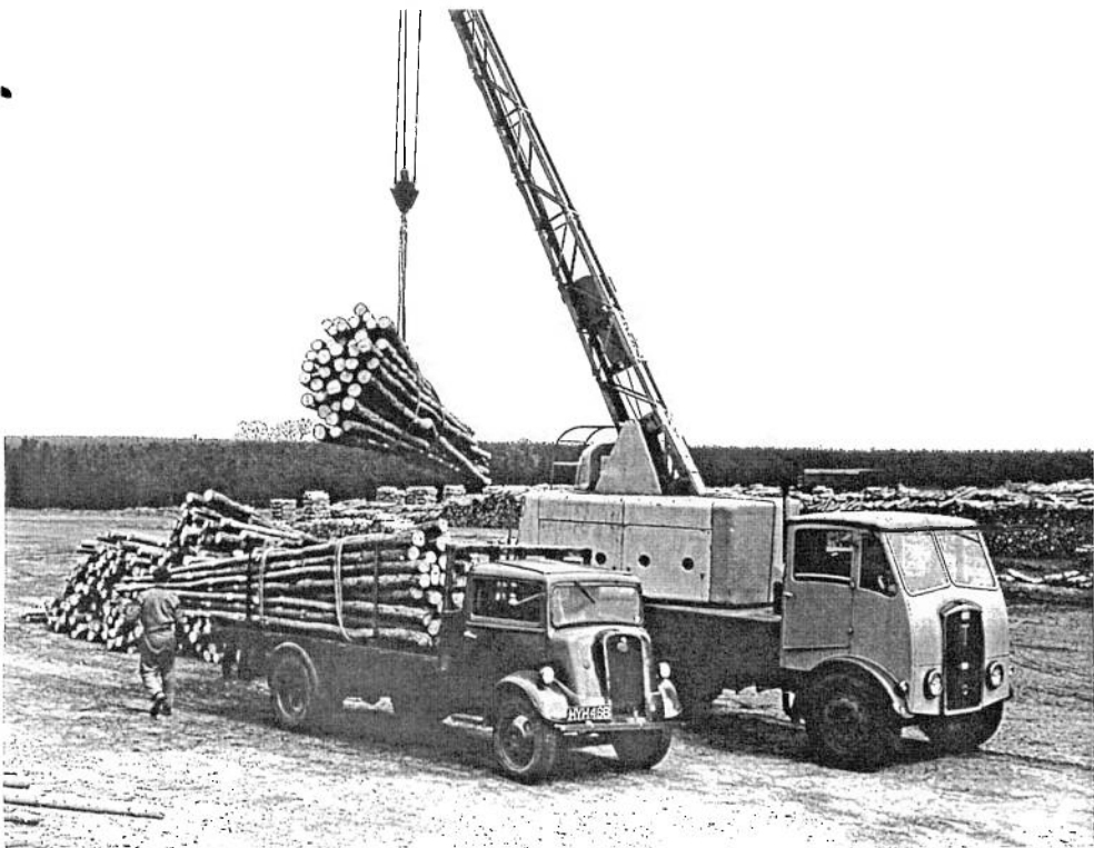
Plate 10. Early Coles crane offloading unpeeled poles using rope slings inserted during loading.
