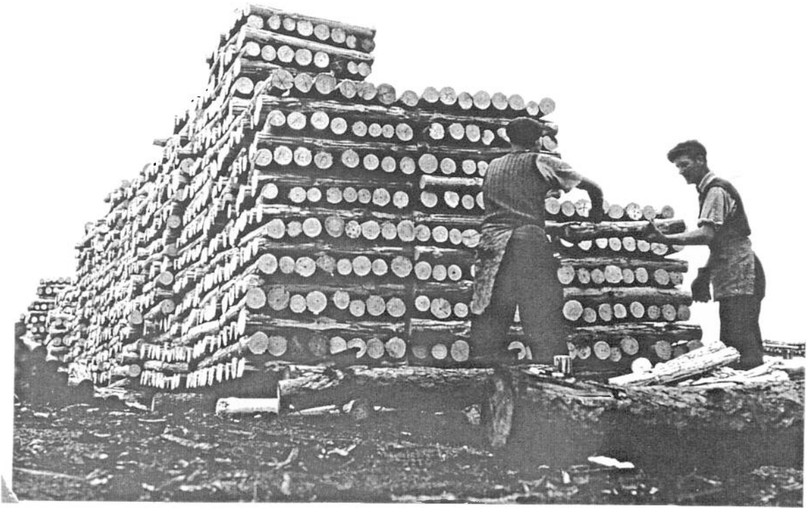
Plate 47. Cross stacking pitprops to improve seasoning early 1950's. Very costly in terms of space.
