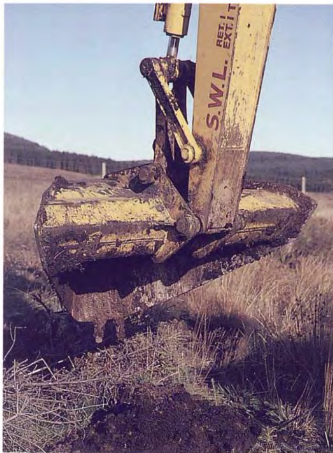
Mound produced by excavator mounding.
