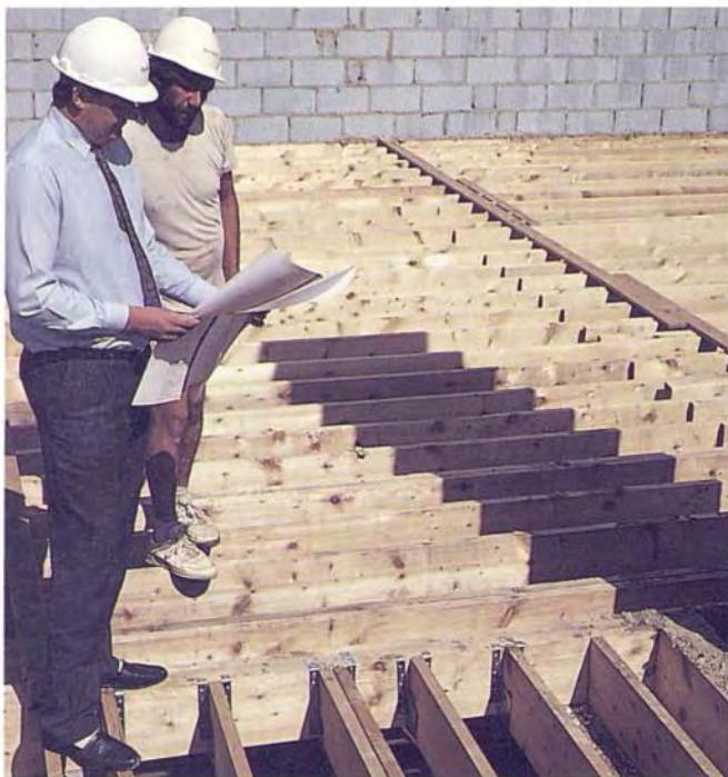
Home-grown softwood timbers used in construction.
