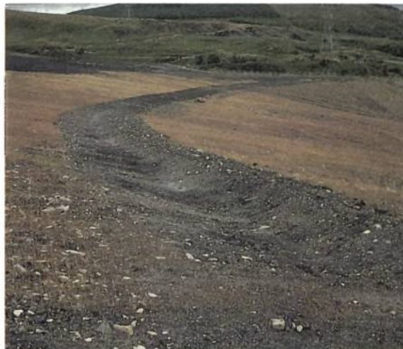
Plate 16 Contour berm on restored opencast coal site, South Wales.
