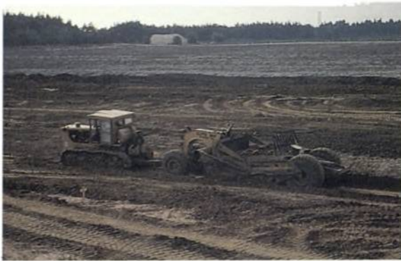
Plate 10 Widespread trafficking by earthscrapers, leading to soil compaction.
