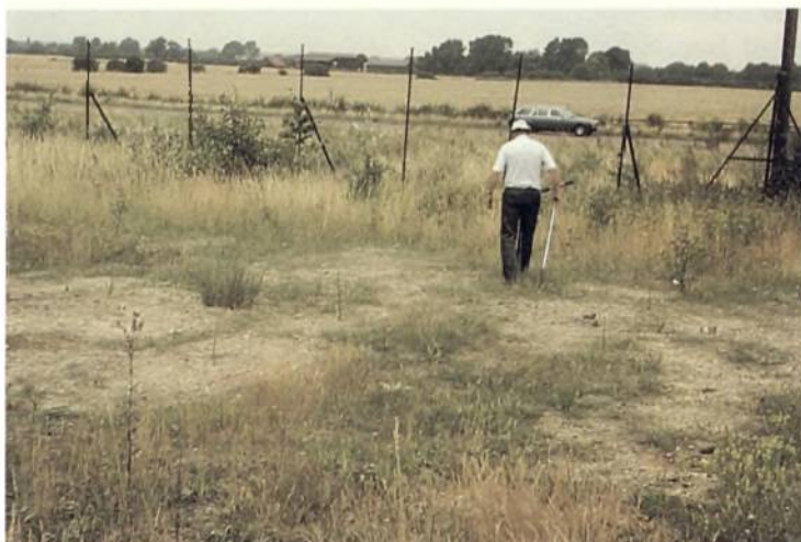
Plate 25 Effect of landfill gas on trees and ground vegetation.
