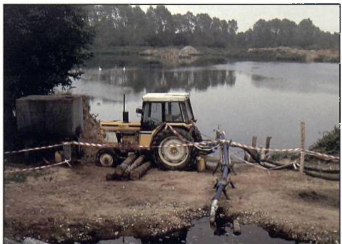
Plate 3 Early pumping system, located between wet store (foreground) and gravel pit (background).
