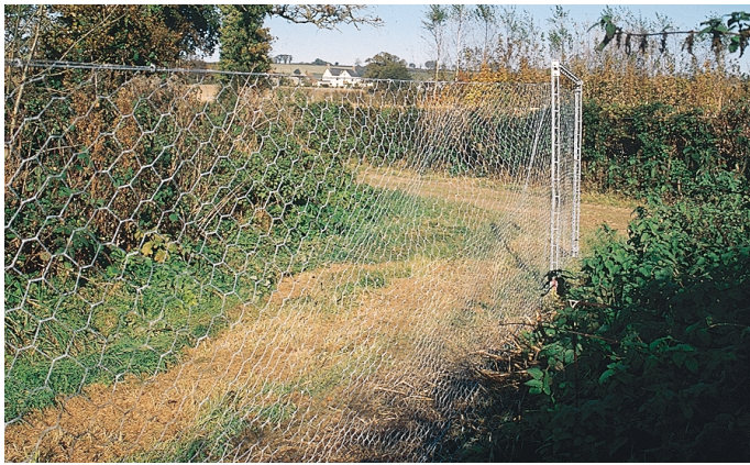
Figure 2 Lightweight hexagonal mesh netting
