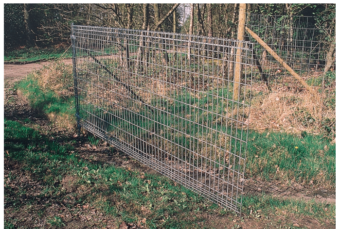
Figure 8 Rolled-top gate hung on T-bars
