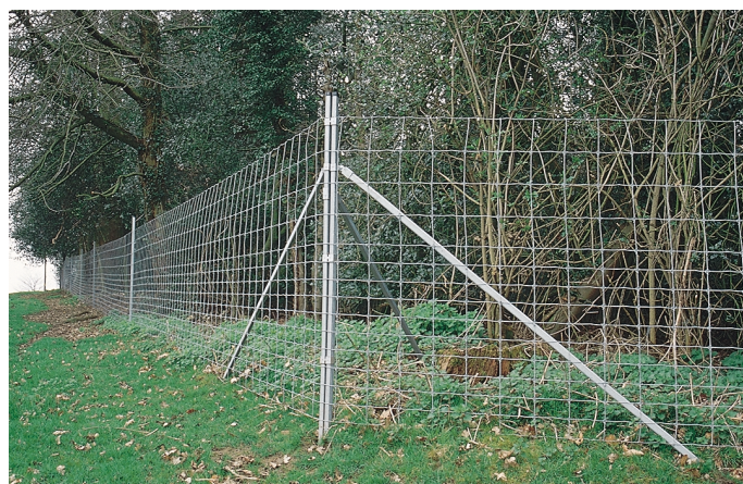
Figure 1 Staplelok post and light HT wire mesh
