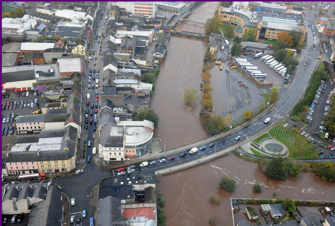
Flooding in Omagh, Northern Ireland, October 2011 (Michael Cooper, DfI Rivers)
