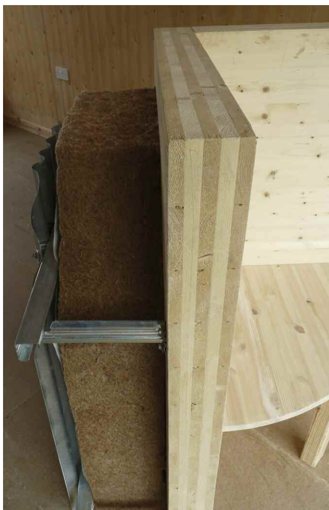
Figure 3.3 Five layer cross-laminated timber panel with insulation and cladding attached.
