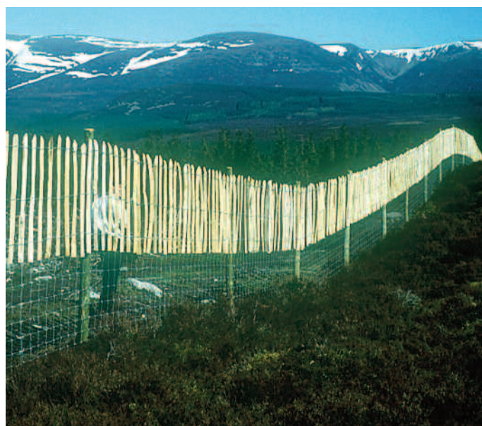
Figure 5b Birds flying at an angle to the fence will see a 'wall' when triangular sawn softwood droppers or split chestnut palings are used.
