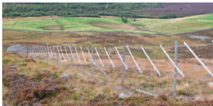
Figure 4c 0.9 m wooden droppers fixed vertically at close spacing.
