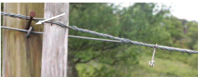
Figure 8c A nail in each stake assists hanging paling rolls.
