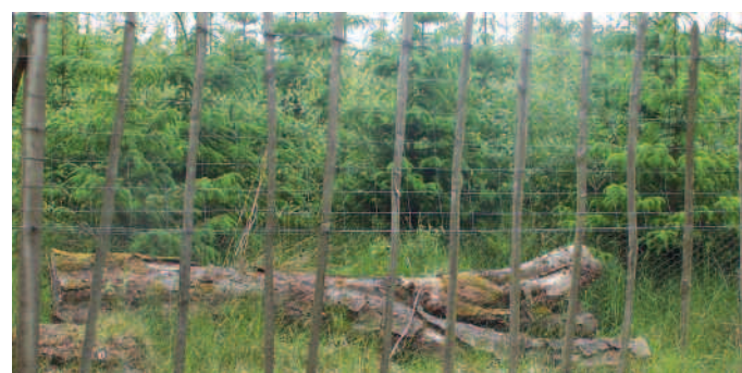
Figure 4d 1.8 m pales fixed vertically at wide spacing.
