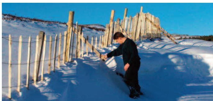
Figure 9c Struts are vital in exposed or known snowfield locations. Creating deliberate 'weak points' in line wires and mesh will mean that only a limited length of fence may collapse during adverse weather.
