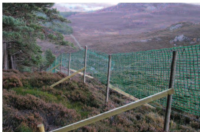
Figure 2c Green netting on a sheltered perimeter fence at the bottom of a glen. Note that extra struts that have been added to the fence.
