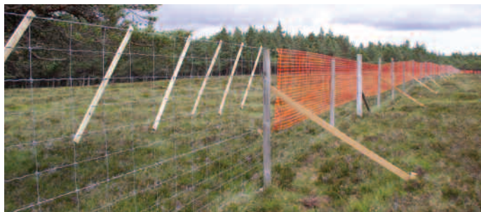
Figure 9b Extra struts added to a newly-marked fence in an exposed location.
