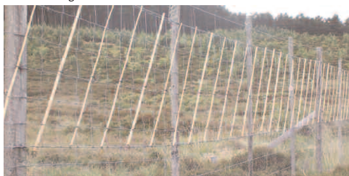
Figure 6 Bamboo droppers are relatively less visible than other fence marking materials.
