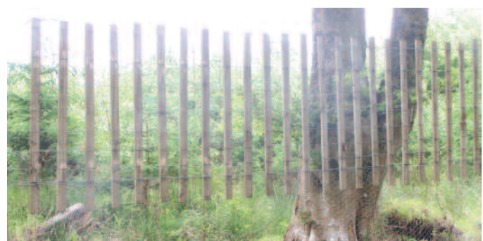
Figure 4c 0.9 m wooden droppers fixed vertically at close spacing.
