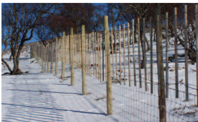
Figure 10 New deer fence comprising wire mesh on the bottom half and rolls of timber droppers on the top half.
