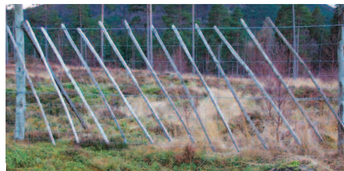
Figure 4d 1.8 m pales fixed vertically at wide spacing.
