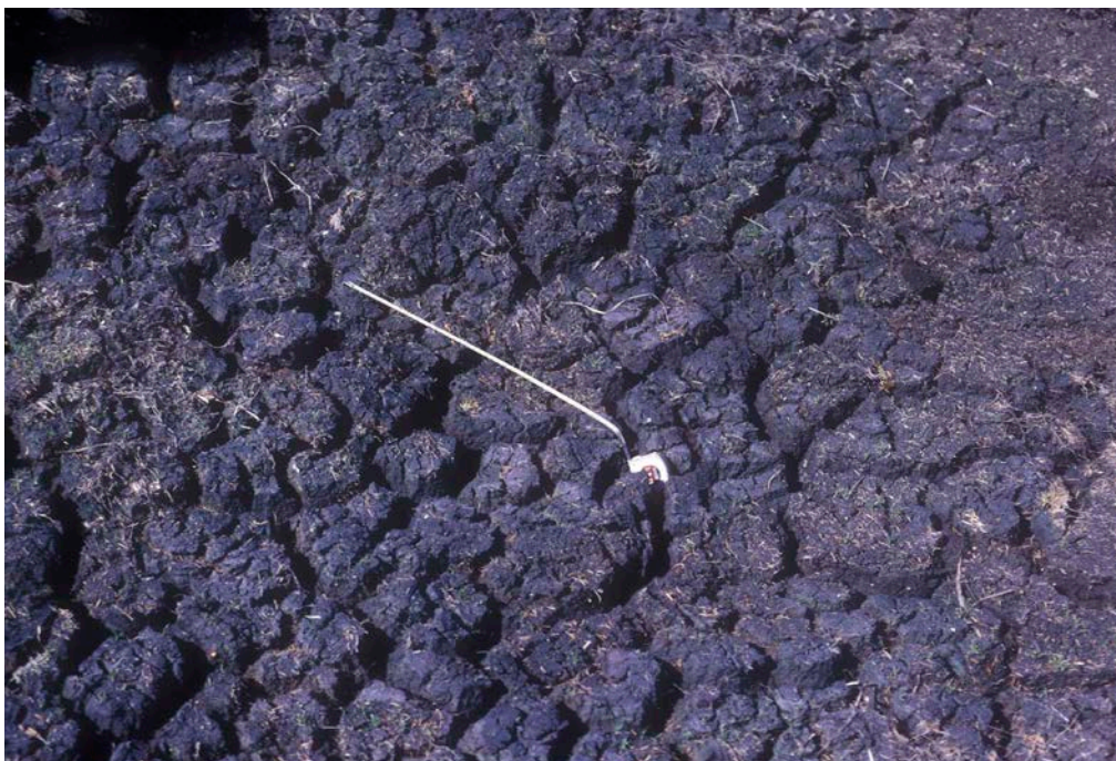
Figure 14 Signs of extensive cracking on peat.
