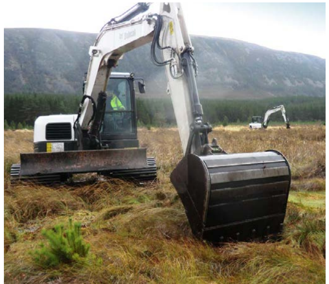
Figure 11 Diggers preparing to block ditches as part of restoration work.
