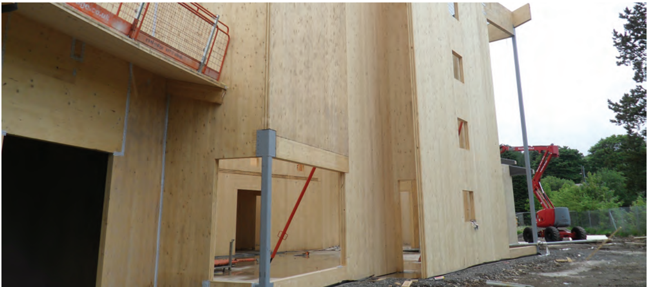
Figure 7 A cross-laminated timber building during construction. Beattock Primary School, Moffat. DGDesign.
