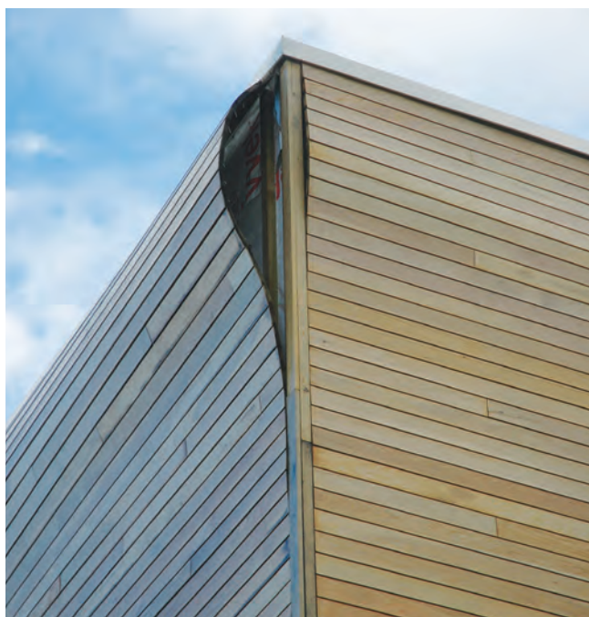
Figure 20 Failure of external timber cladding due to the boards being installed with inadequate expansion gaps.
