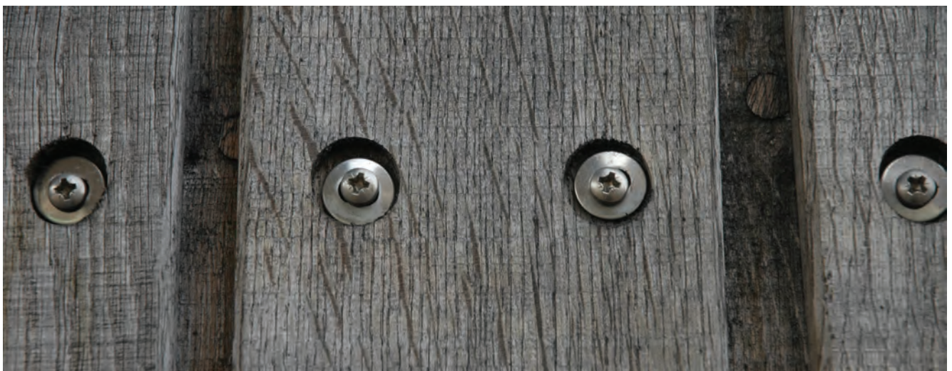
Figure 25 External cladding of green oak detailed to accommodate shrinkage as the timber first dries.
