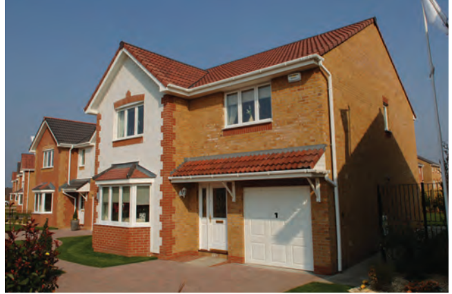
Figure 6 A typical timber-framed house with masonry cladding.
