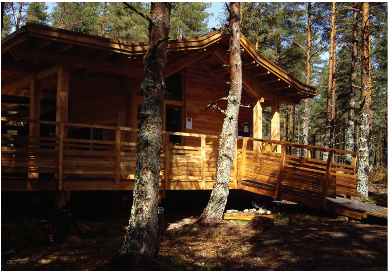
Figure 43 Strathnairn Shelter near Inverness uses a post-and-beam construction formed from local timber. Neil Sutherland Architects.
