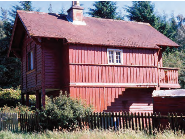
Figure 35 Completed in 1834, Swiss Cottage near Fochabers is believed to be the oldest surviving timber-framed and -clad house in Scotland. It was built using local plantation grown Scots pine; the timber was not preservative treated. Buildings such as this suggest that the desired service life values quoted in Table 16 considerably underestimate the performance that can be achieved in practice.
