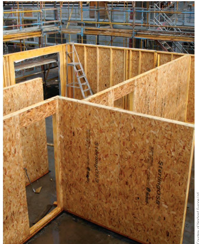
Figure 3 A timber-framed building during construction.
