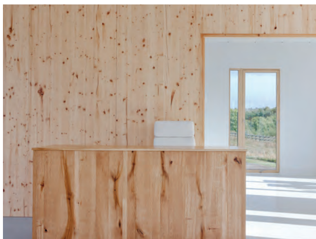
Figure 11 Prototype cross-laminated timber shearwall made of UK spruce at the BRE Innovation Park, Ravenscraig. Kraft Architecture.
