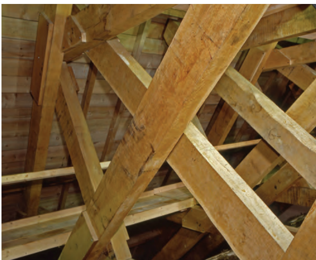
Figure 41 Visually graded oak used for new roof trusses over the south transept of York Minster. Ove Arup & Partners.
