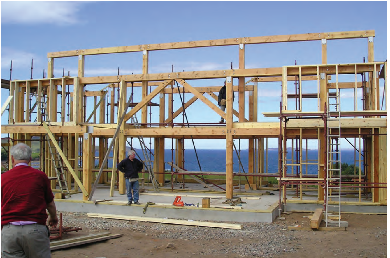
Figure 4 A post-and-beam building during construction.
