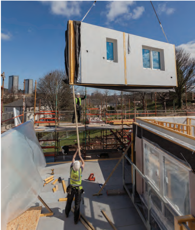
Figure 5 Delivery of a prefabricated timber frame wall panel to site.
