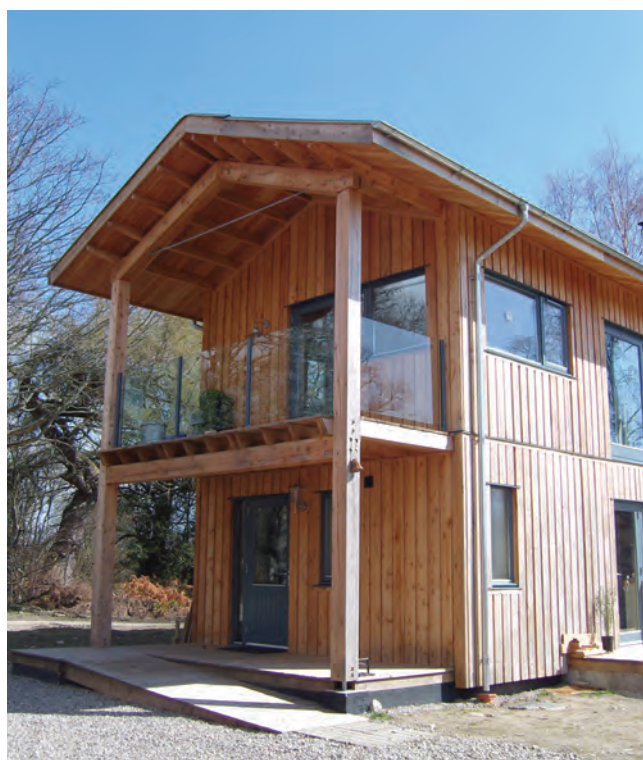
Figure 13 This house near Alness in the Scottish Highlands illustrates the floor span that can be achieved using readily available softwood joists. Neil Sutherland Architects.
