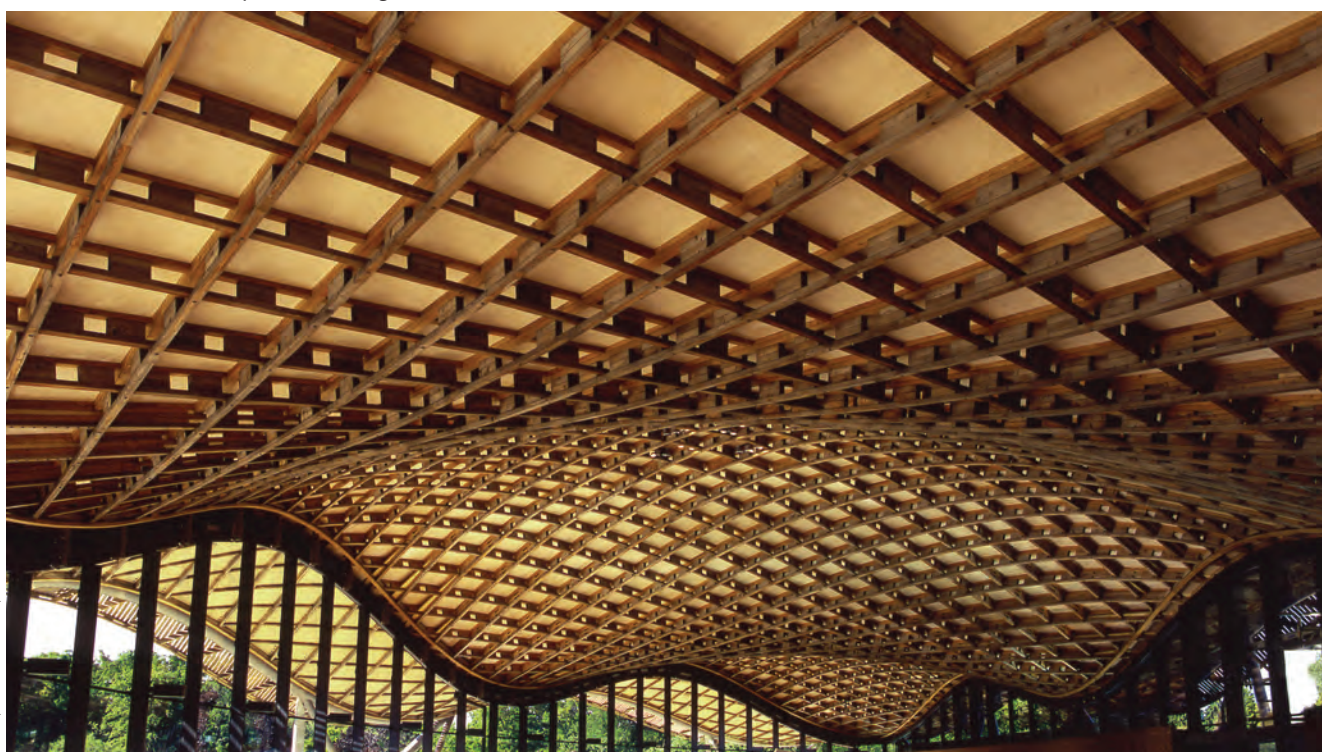
Figure 12 Gridshell roof of the Savill Building by Glenn Howells Architects. Over 20 kilometres of finger jointed larch battens were used to form the four layer structural grid.
