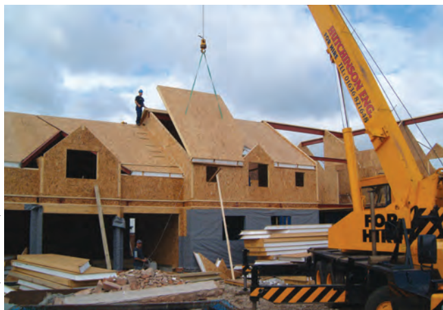
Figure 18 Structural Insulated Panels (SIPS) being used to construct walls and roofs of a housing development.
