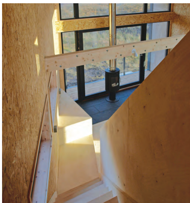
Figure A5.3 The walls of this timber-framed house on Skye are lined with UK produced orientated strand board. Rural Design Architects.
