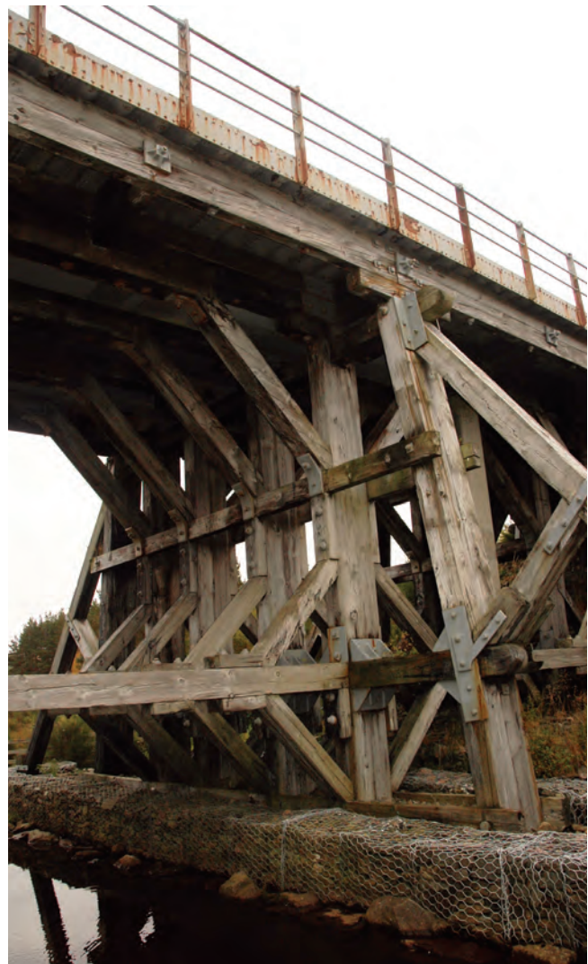
Figure 38 Aultnaslanach Railway Viaduct at Moy near Inverness was completed in 1897 and is the only surviving structure of its type on a main railway line in Scotland and possibly in Britain. The trestles are made from imported pitch pine and have been preservative treated.
