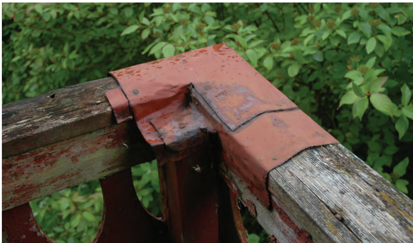
Figure 42 Mitre joints can act as a water trap in use class 3 and so are prone to wet rot.
