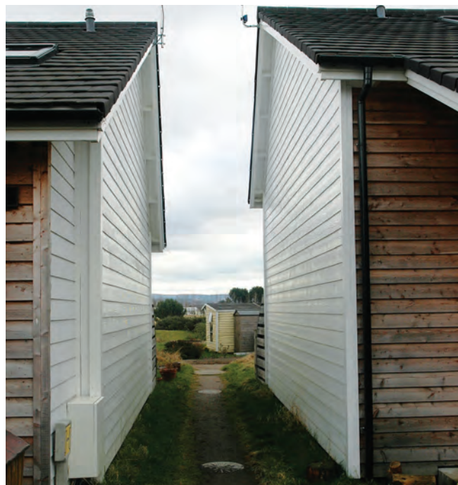
Figure 33 Fibre cement cladding has been used on these gable ends. This is because Scottish Building Standards do not permit combustible cladding on facades that face onto an adjacent ownership boundary.
