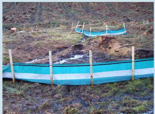
Figure 34f Use timber posts at a slight upslope angle to support longer lengths of geotextile barrier. Consecutive barriers, as shown here, may be needed to manage a sediment pollution incident.
