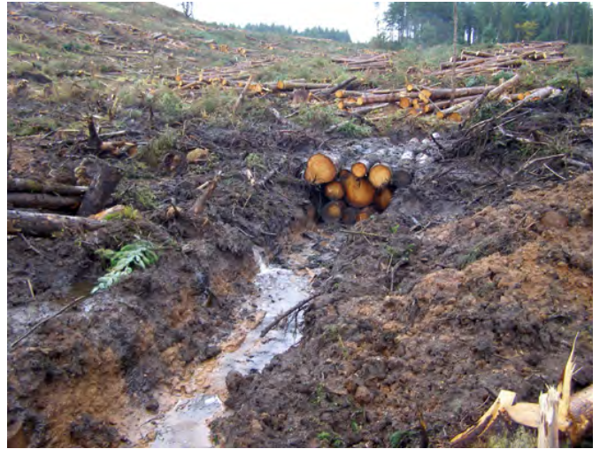
Figure 29 In this situation pipes need to be installed along with logs to prevent water backing up and causing site waterlogging and ground damage.
