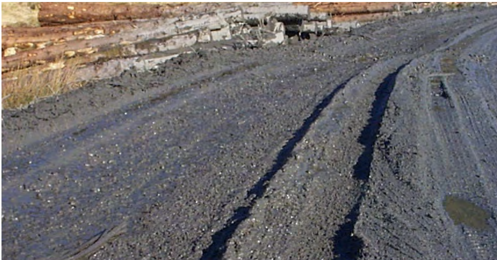
Figure 15 Damaged road surfaces can quickly degrade and cause pollution through sediment run-off.
