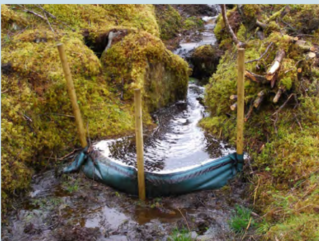
Figure 34e Terrain fabric can be used to create a small silt trap but is readily bypassed by significant flows.
