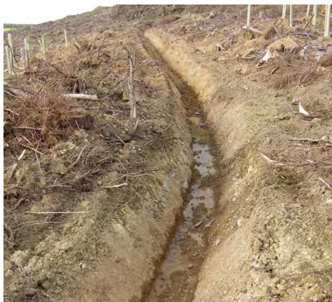
Figure 9 An example of a well-designed cut-off drain controlling restock site run-off.
