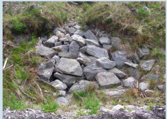
Figure 34d A collection of different sized stones can provide an effective drain-end sediment trap.
