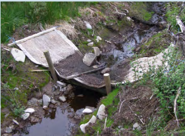
Figure 34c Coir matting can help trap fine and coarse sediment across a range of flows.
