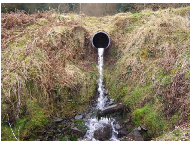
Figure 17 Hanging culverts should be avoided, especially in fish-bearing streams.
