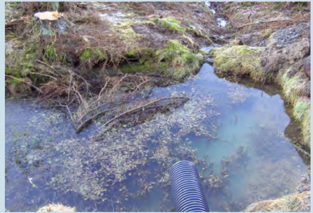
Figure 34b An example of a poorly designed silt trap: culvert aligned with outflow, promoting slip-streaming, while hanging inflow will generate turbulence and stir up sediment.
