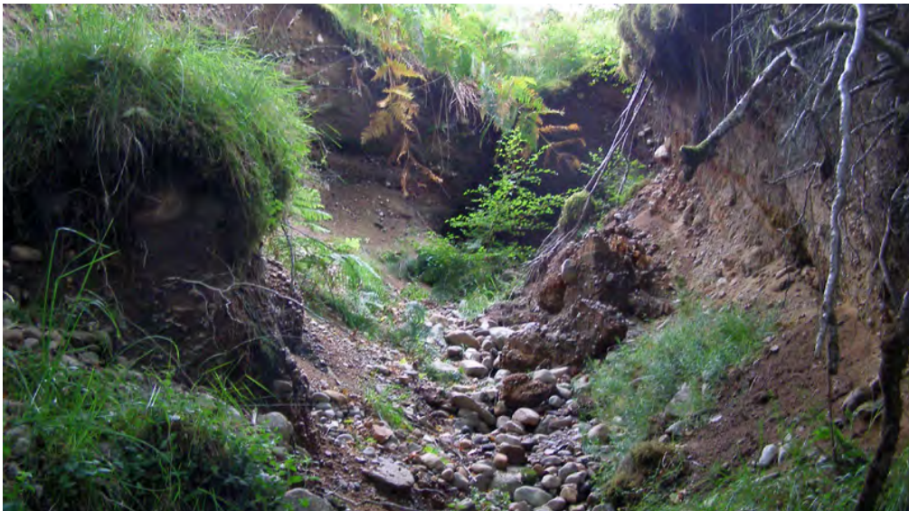
Figure 7 Excessive run-off has caused major erosion and gullying within this drain.
