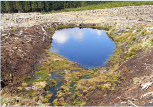
Figure 34a Large silt traps can hold more water and help to settle finer sediment but need care to avoid washout of bund, especially at outlet at high flow.
