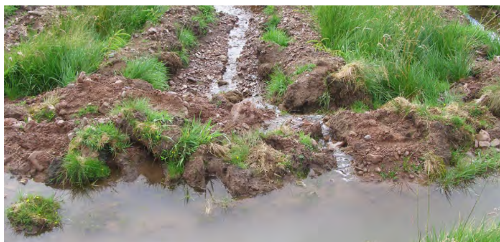
Figure 36 Heavy rainfall has resulted in water overspilling from a drain into a lower cultivation channel, causing erosion and turbid water discharging into a watercourse.
