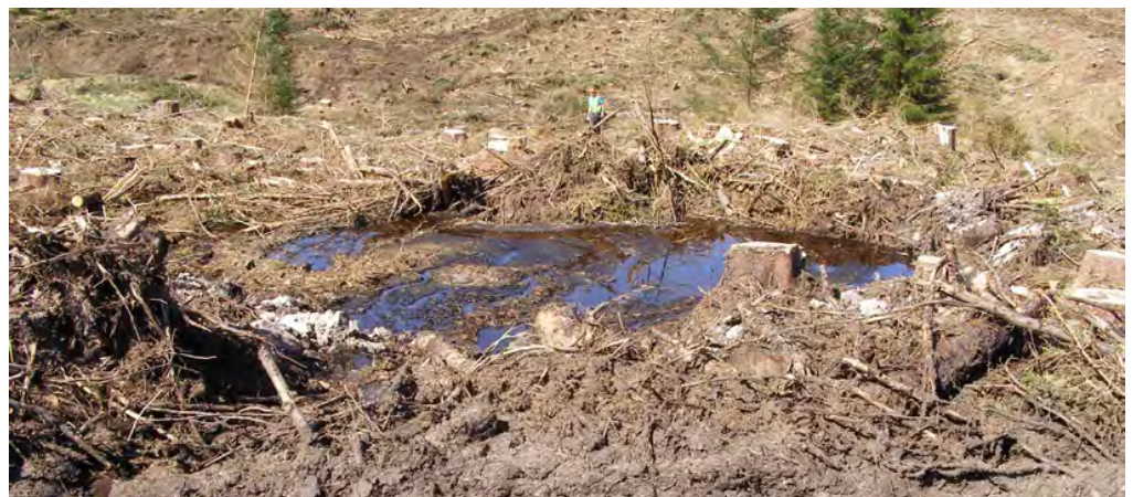
Figure 33 A brash bund can provide an effective filter for retaining sediment, providing run-off volumes do not exceed the capacity of the system.
