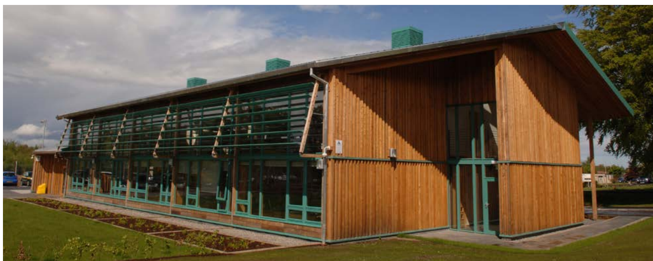
Figure 3.3 This Forestry Commission Office at Smithton in Inverness is clad with furfurylated home-grown Scots pine (Jardine, 2010).
