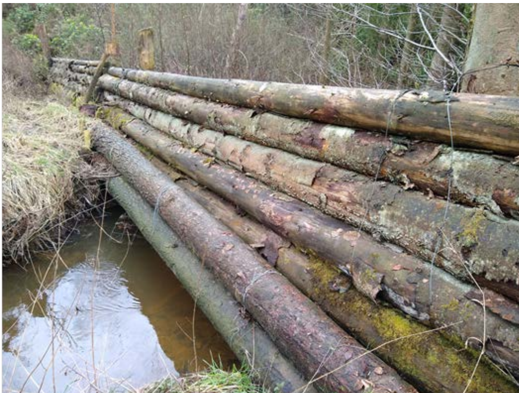
Figure 6 Image showing the timbers spanning the river channel on the lower bund, with the most decayed log covered by moss (fifth timber down from the top). The two bottom timbers (numbers -1 and -2 in Figure 4) were replaced in 2019 and therefore much less degraded.
