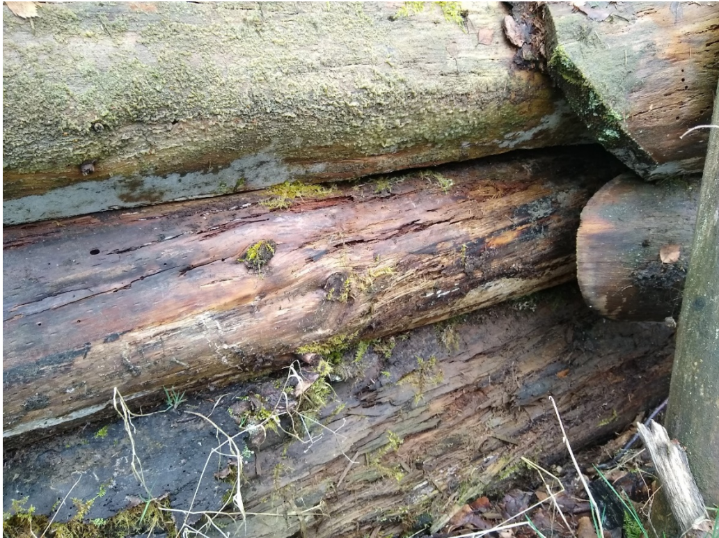
Figure 7 Close up image of decayed timber at the 18 m junction on the downstream flood storage bund.
