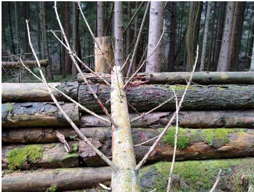
Figure 9 Image of the decaying timbers at the junction at 27m from the left edge of the upstream flood storage bund, partly damaged by the windblown tree falling onto the structure.
