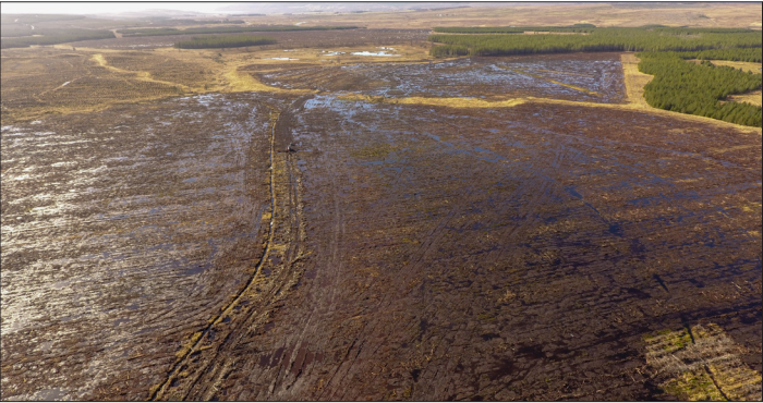
Rewetting afforested blanket bog at Dalchork Forest in the north of Scotland. An excavator turns the stumps over into the plough furrows, then runs across the ploughing, pressing them down. Vegetation regrows quickly on the flat, wet surface.
