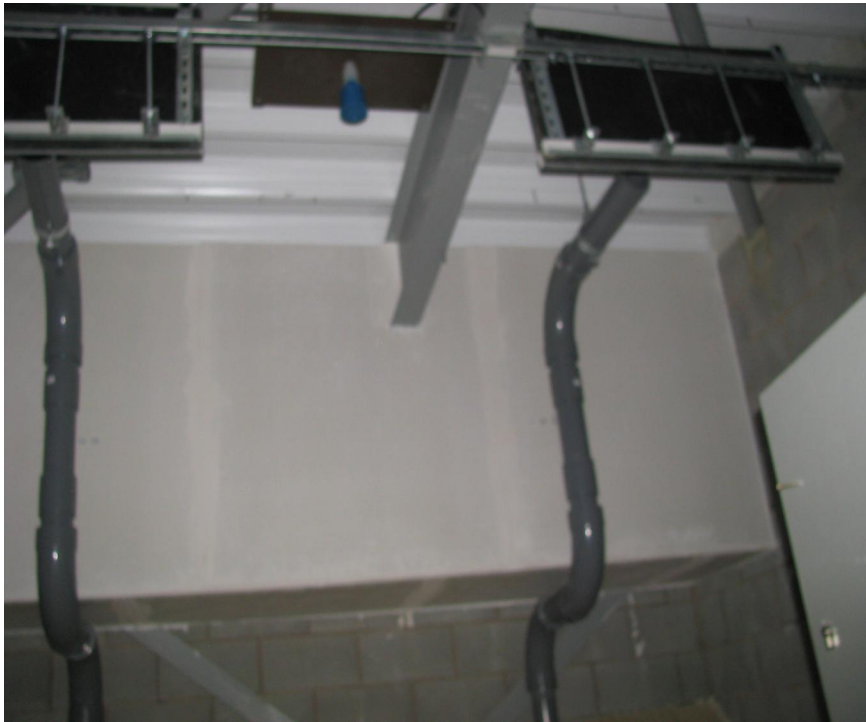
Twin Pellet Delivery Pipes with Impact Cushion Mats. The mats are too close to the pipes and will reduce the filling capacity of the silo
