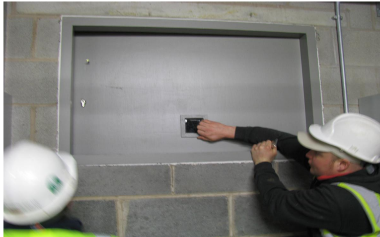
High Level Access Door to Silo
