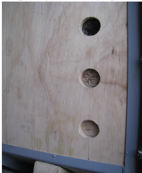
Figure 1 – Pellet Level Sight Windows
