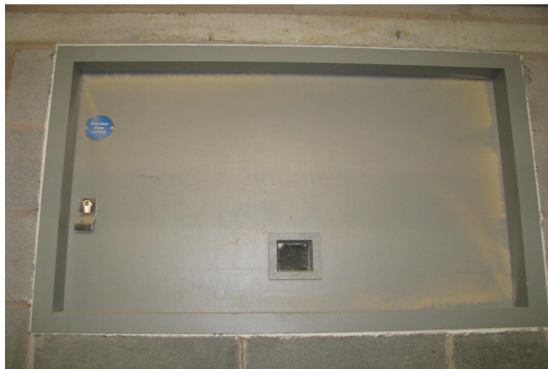
Emergency Access Door to Silo with sight Glass. Door not properly sealed so allowing dust to escape. It opens internally to silo which prevents access when silo is full and the sight glass is too small to be useful.
