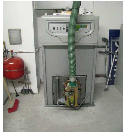
Pneumatic delivery system – with poor design pellets can bridge and cause blockages
