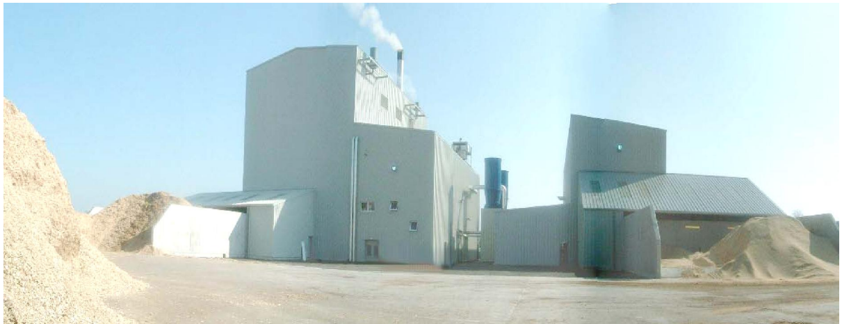
Balcas 55,000t/yr Pelletising and CHP Plant, Enniskillen
