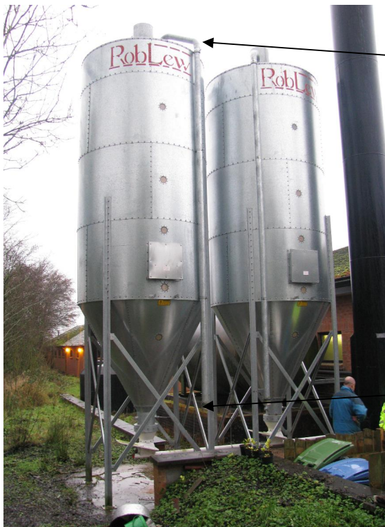
Tall pellet silos need a vertical fill pipe and soft bend at the top
