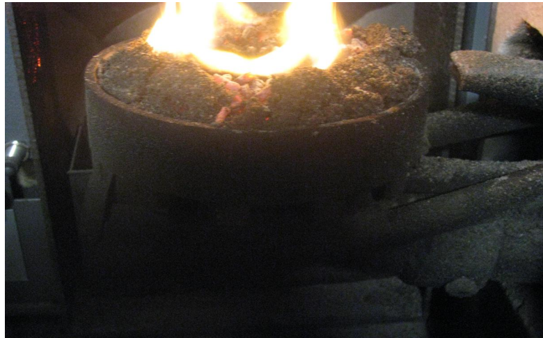
Damp pellets, poor quality pellets and/or poor combustion causing clinkering
