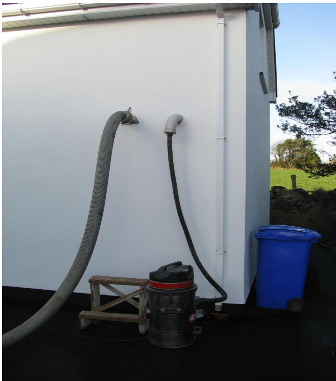
Pellet Delivery into Pellet Silo with Dust Extraction
