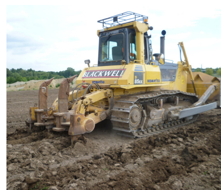
Figure 1 Subsoil ripping using tracked machinery (Photo: © Tim O'Hare Associates)
