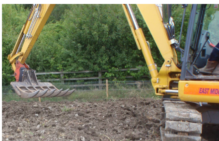
Figure 7a Topsoil cultivator – tracked excavator with landscape rake attachment.
