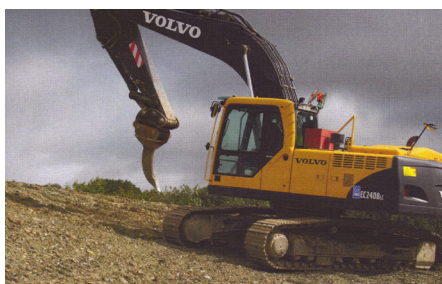
Figure 4a Tracked excavator with a single rigid tine.
