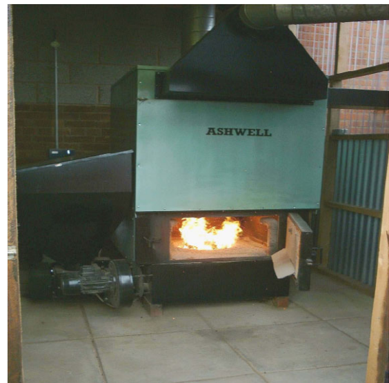
Figure. 2 Ashwell Compac air heater unit firing wood pellets
