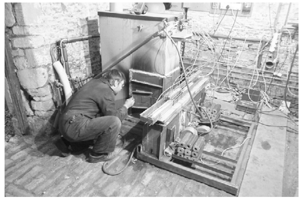
Figure 1 Final configuration of cartridge burner installation at Overmoor farm
