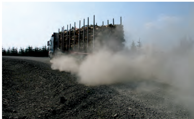
Figure 8 Blow-away of dry road material.
