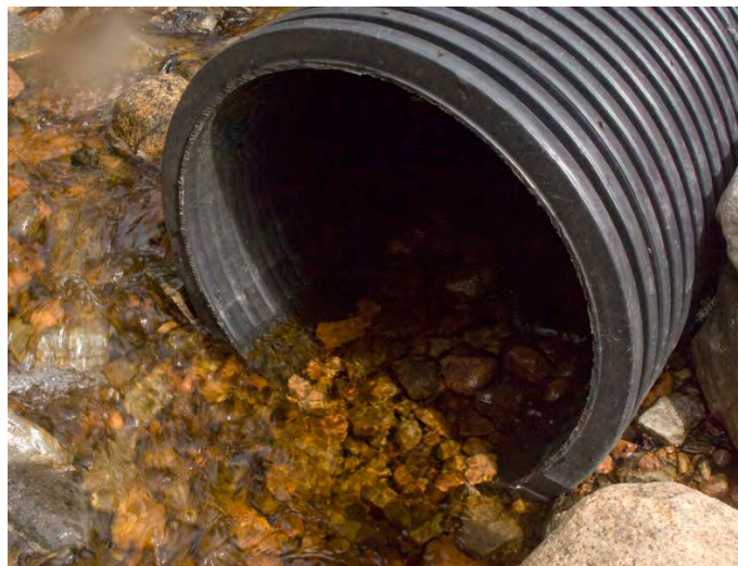
Figure 10 A plastic culvert under a forest road.
