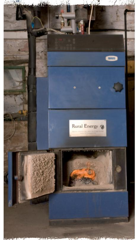
The boiler itself might cost around three times the price of a top end gas boiler, and most will require in addition a pellet store, pellet feed mechanism and a flue. Some are available with a built in hopper that requires periodic filling from a bag. Small systems tend to be significantly larger than the equivalent capacity gas boiler as a ceramic lined firebox is required as well as mechanical components to feed the solid fuel.
