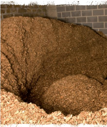
However this corresponds to about 5.5 tonnes, which may be around the minimum delivery quantity of a commercial supplier, and would require a bespoke chip store of at least 30m<sup>3</sup> capacity. The cost and space required for this tends to be beyond the scope of most domestic installations. It can represent a very cost effective, low carbon option for larger buildings, hotels, leisure centres, and businesses with sufficient storage space.
