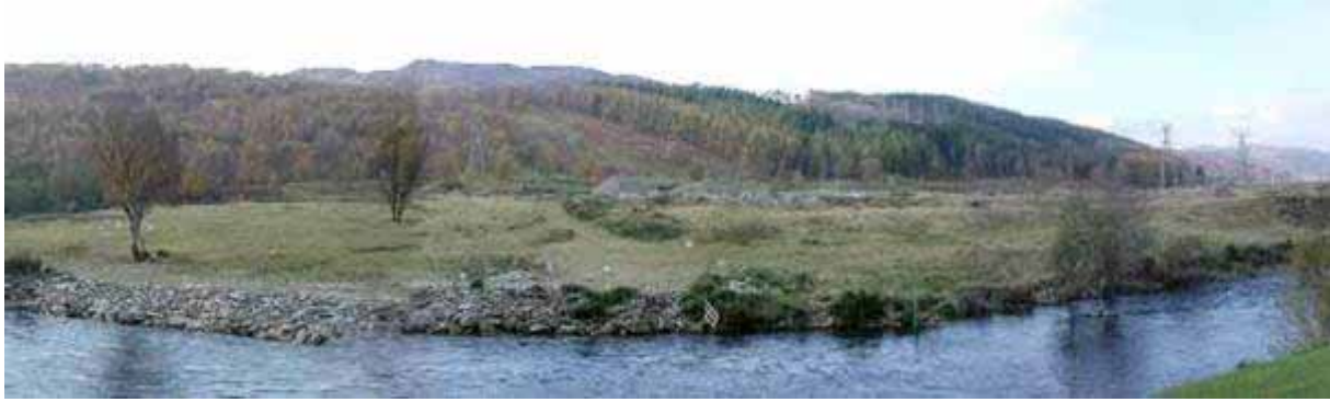
Fig 8.5 Kerrow from Fasnakyle Power Station
