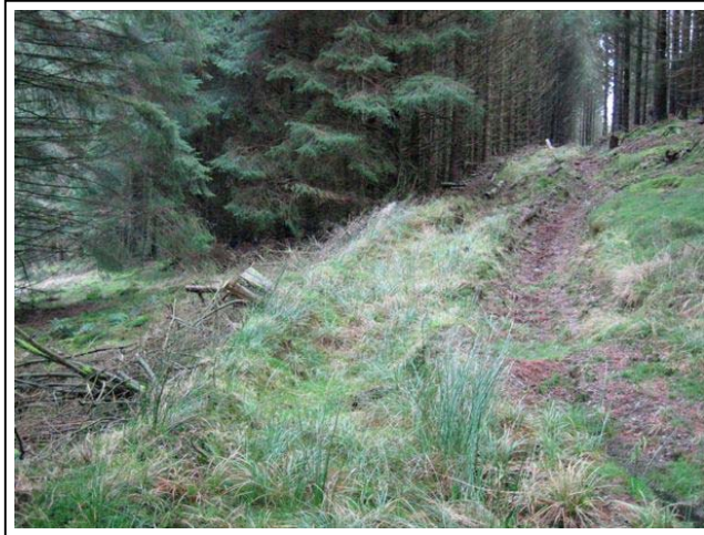
Figure 34 Inverted stump and brash formation to allow machine movement over steep cross slope
