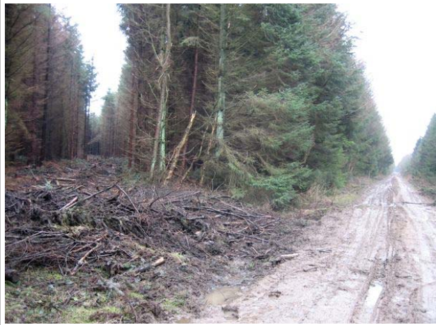
Figure 8 Brash 'key route' constructed at an acute angle to main forest road
