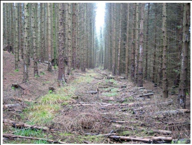
Figure 30 Corduroy rack formation, constructed from brush and chip wood specification produce
