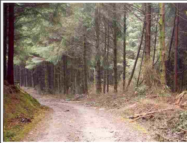
Figure 31 Brush access track constructed adjacent to metalled forest road preventing damage to the metalled road
