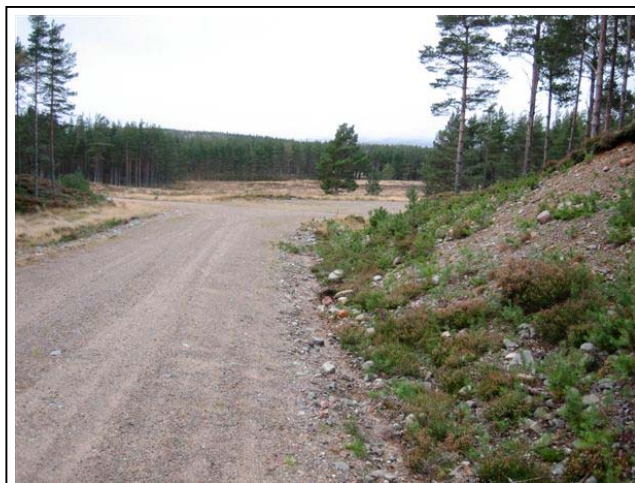
Figure 50 Forest road constructed from locally won stone, note natural regeneration on disturbed bank adjacent to road
