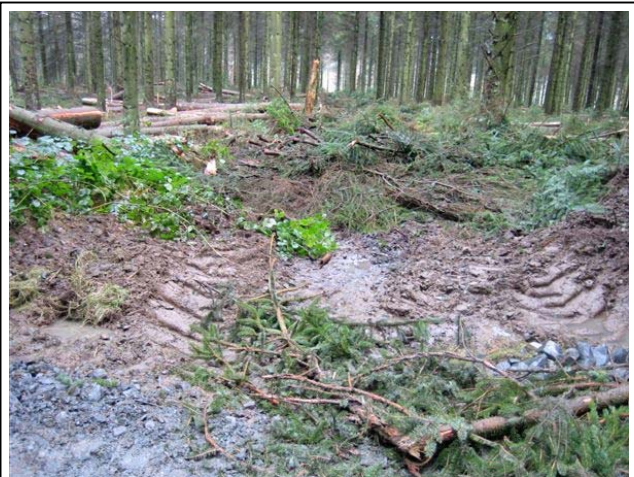
Figure 24 Soil disturbance can occur between the stone-surfaced secondary road (foreground) and brash-surfaced rack (background). The proposed solution to preserve the entrance to the rack is to stone the rack bell-mouth safeguarding the condition of the rack into perpetuity
