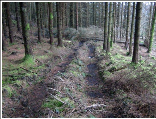
Figure 29 Travelled rack without corduroy rack construction showing rutting
