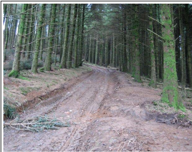
Figure 12 Cut-off drain viewed from down-slope
