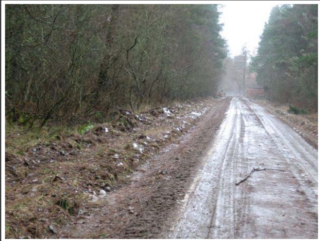
Figure 60 Harvester and Forwarder movement adjacent to the road, preserving the road surface condition for timber lorry travel
