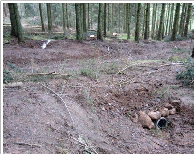
Figure 11 Well constructed culvert, instated prior to harvesting through consultation with FC Civil Engineering
