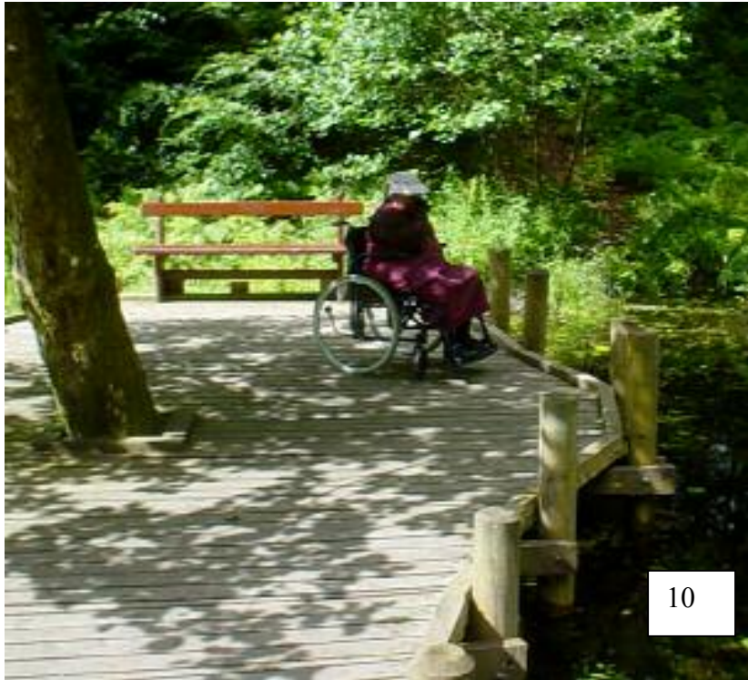
Figure 10: boardwalk provides access to pond, posts act as trip rail for visually impaired, seat to rear would benefit from arm rests.
