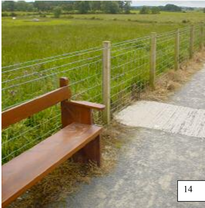
Fig 14: textured concrete indicating position of seating for visually impaired
