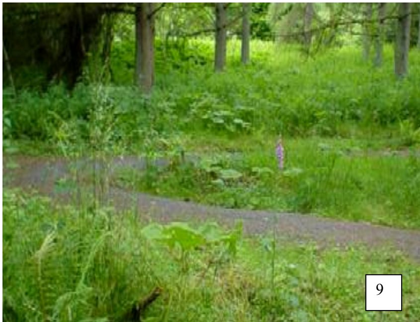
Figure 9: gradient controlled with zig-zag to path
