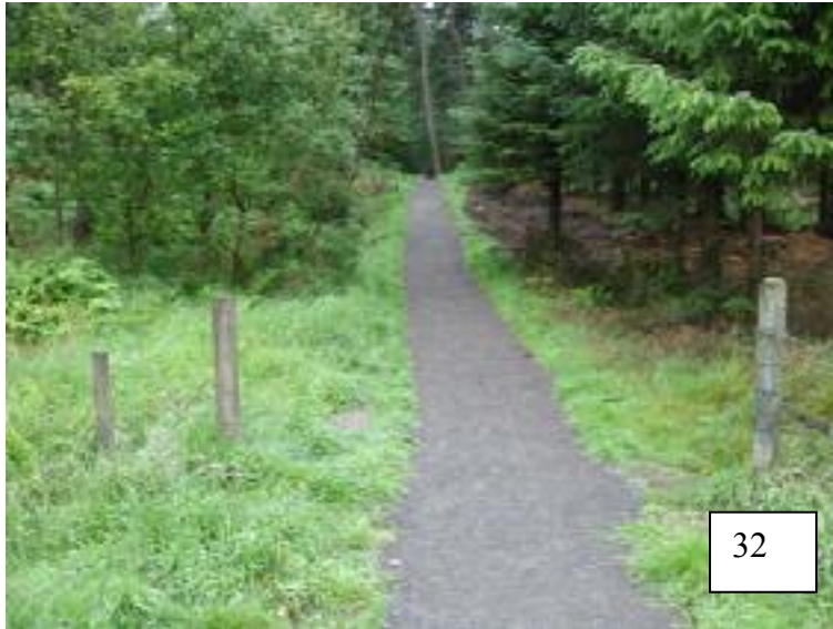
Fig 32: Path construction to BT Countryside for All standards: low gradients, smooth but firm surfacing, and straight.
