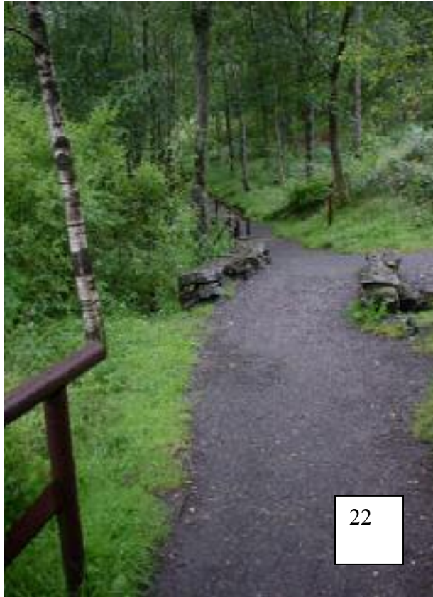
Fig 22: good provision of hand rail to trail but this needs to be continuous along route
