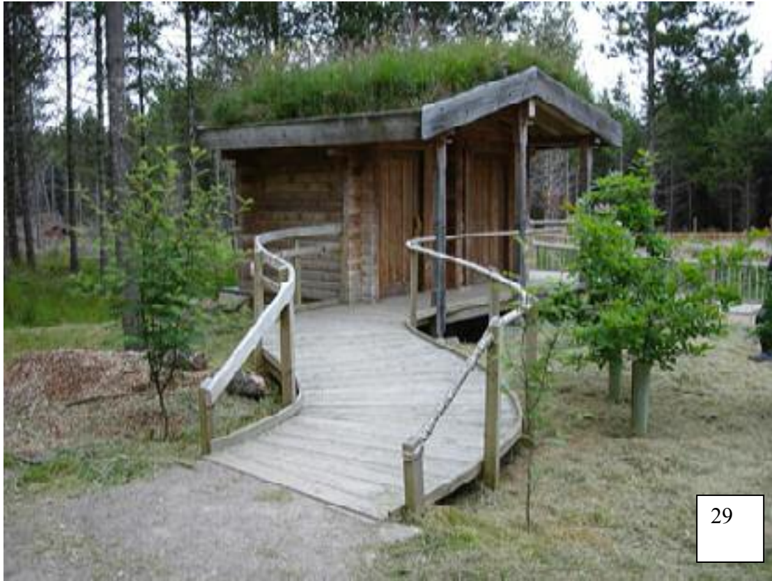
Fig 29: Composting toilets with attractively designed ramps
