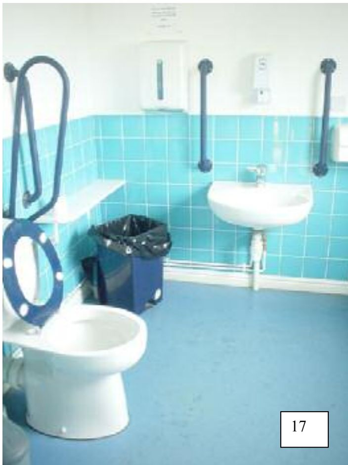
Fig 17: good colour contrast to disabled toilet and good provision of shelves & handles.
