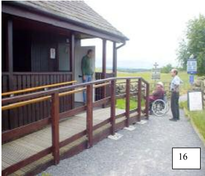
Fig 16: toilet access highly visible and in prominent location
