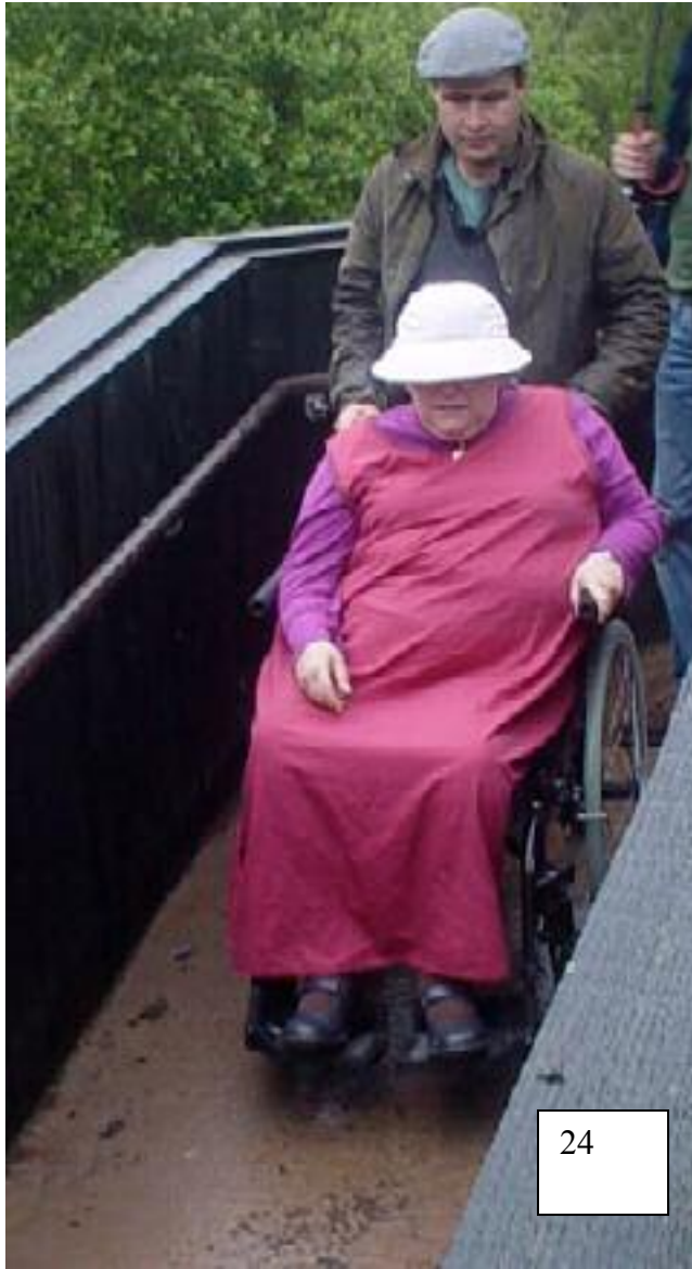
Fig 24: greater colour contrast required between brown handrail and black painted posts.
