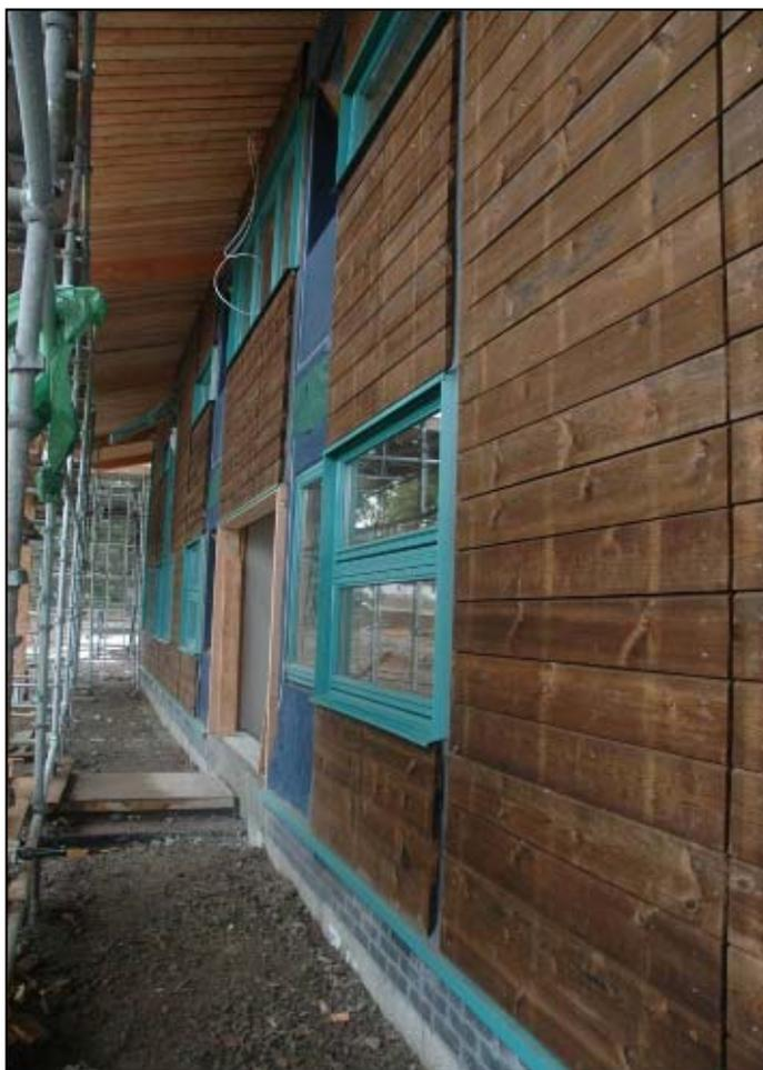
Fig 7. The cladding on this building has been made from Scottish grown Scots pine which has been Furfurlated in Norway. This was a demonstration project but if chemical modification could be developed using UK timber there would be considerable commercial interest.
