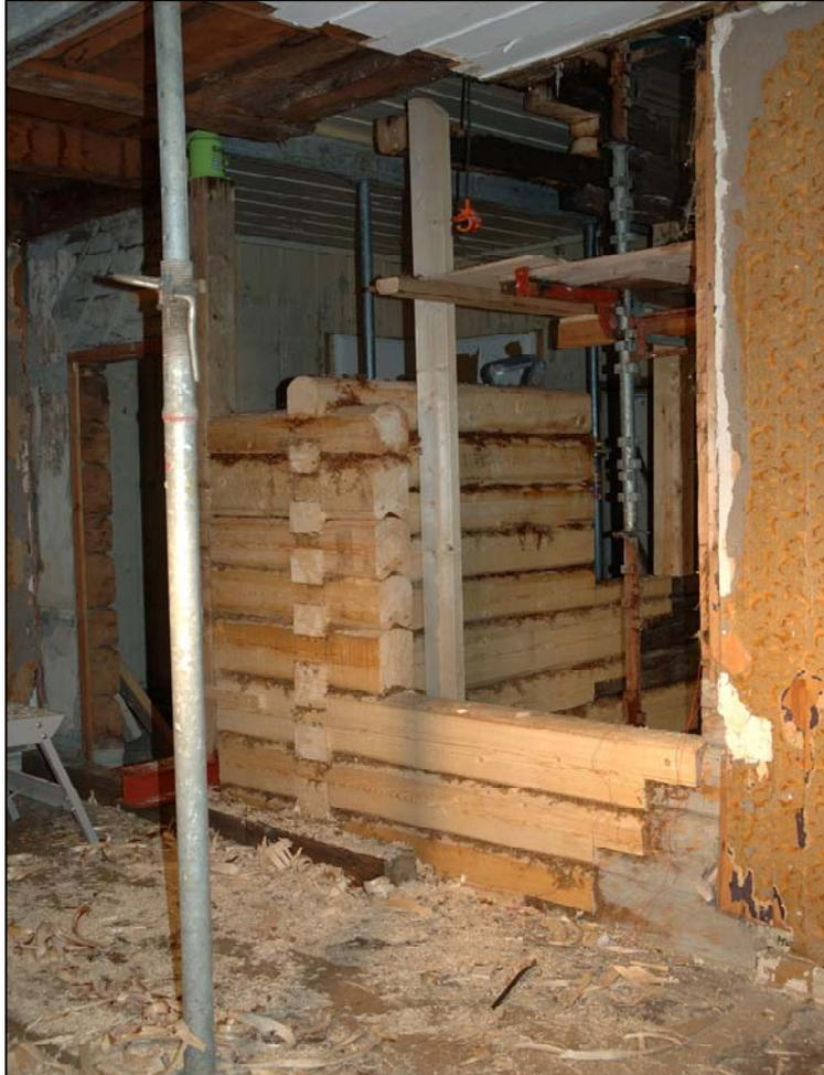
Fig 3. This Norwegian log building is being restored using traditional techniques which include removal of all sapwood
