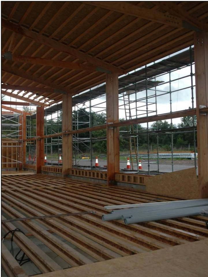
Fig 2. An office building near Inverness built largely from local timber.
