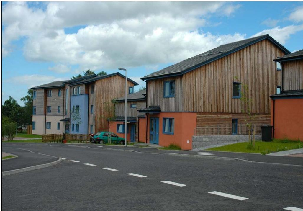
Fig 5. Scottish grown larch used to clad a housing development near Inverurie
