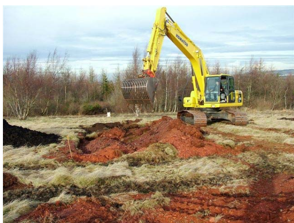
Plate 1. Hitachi PC210LC excavator
